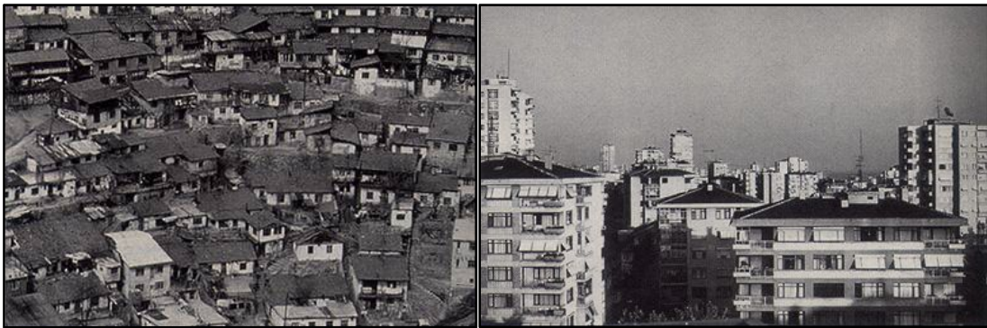
Figure 4.5. Gecekondu and apartments in Istanbul
