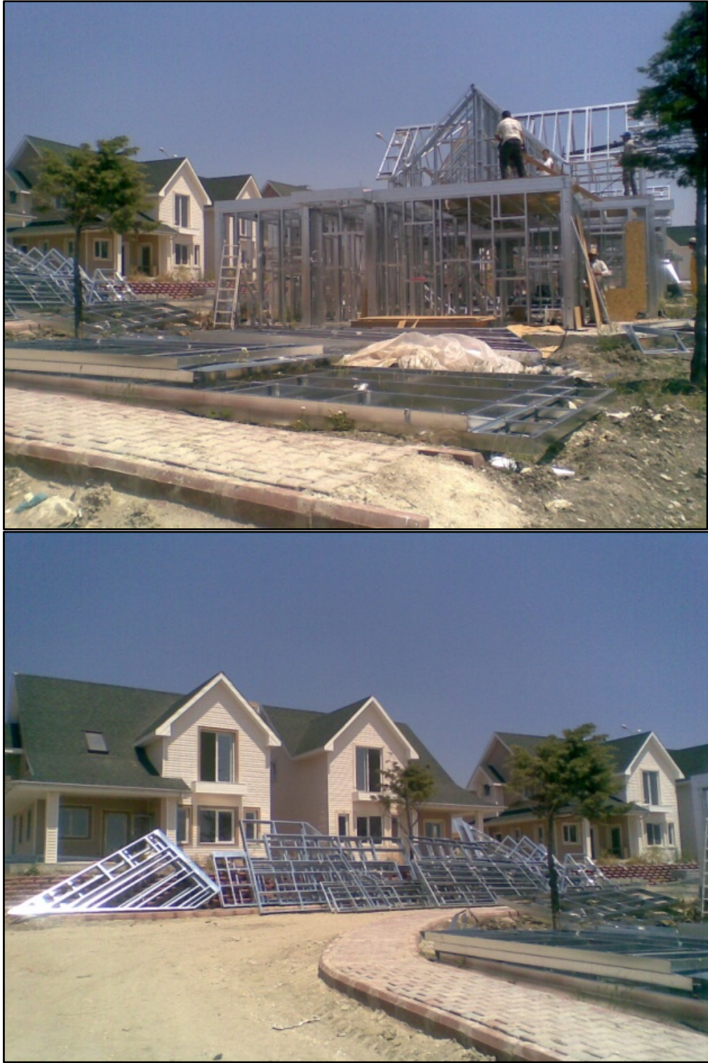
Figure 5.37. Steel Framed Zeytinsuyu Tepesi Houses (Source: Author's archive, June 2008)
