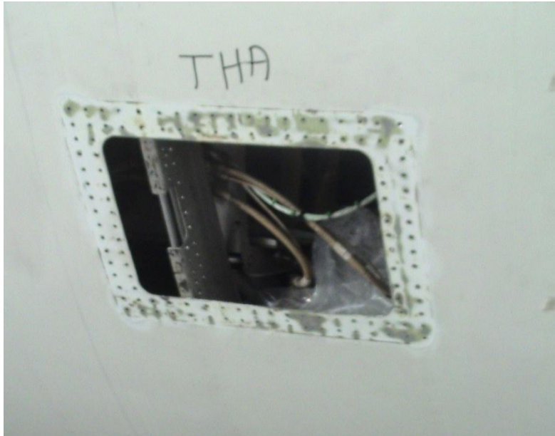
Figure 6.2 Cut-out of the Damaged Skin
