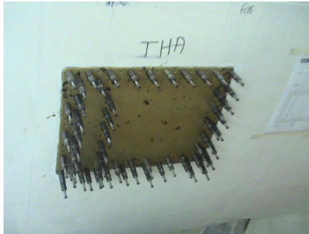
Figure 6.9 Installation of the Fasteners
