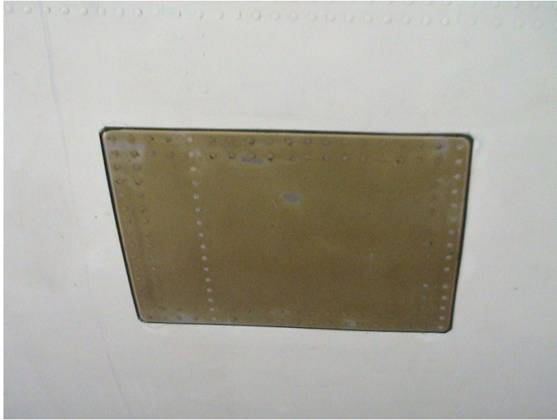
Figure 6.13 Removing of the White Duct Tape
