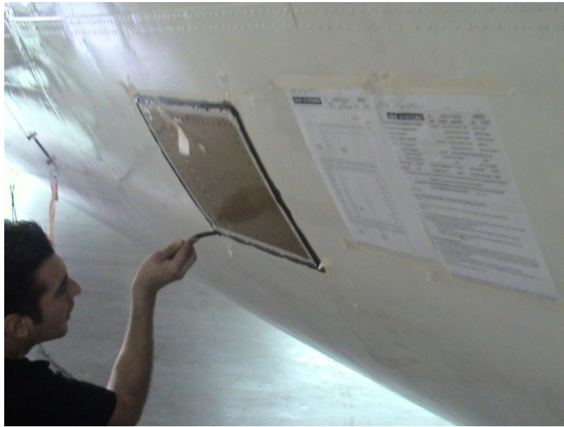
Figure 6.11 Sealing all the Edges of the Doubler with Sealant (Corrosion Inhibiting Brush Consistency)
