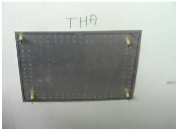
Figure 6.8 Fixing the Doubler
