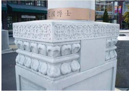
Figure 2.4. SCC enables large variety for formwork designs [11]
