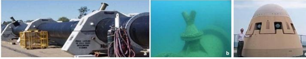
Figure 4.11 : Some examples of multiport discharge outfall constructions, a) alternating diffuser (WaterUse, 2011), b) T-shape diffuser (CEDEX), c) rosette type diffuser (Roberts et al., 2010).
