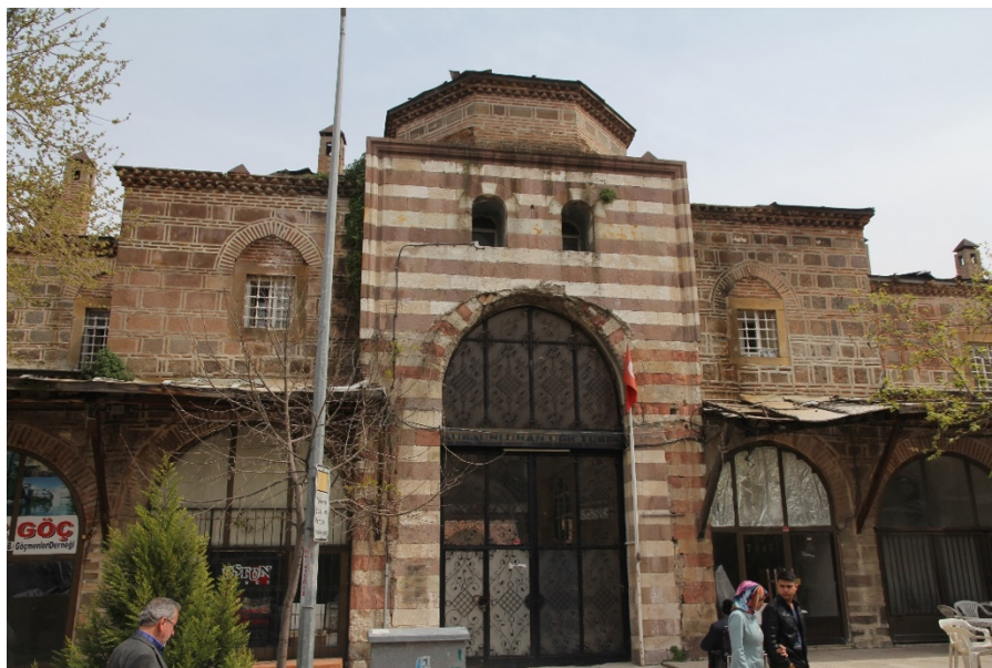
Figure 26. Photo showing the two-color application of stonework at the main entrance.
