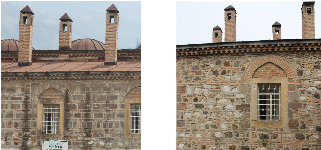
Figure 25. Partial photo of the North (left hand side) and South (right hand side) facades in which masonry works can be easily distinguished (Source: Saygı 2015).
