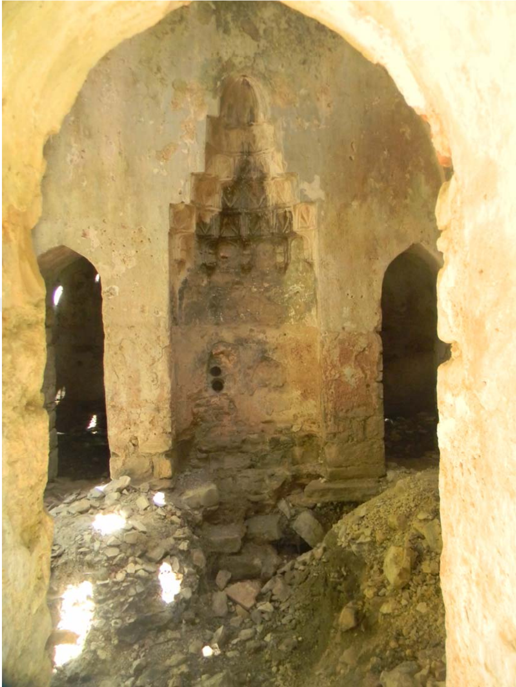
Figure 3.4. Muqarnas decorated fountain niche in the main sıcaklık space
