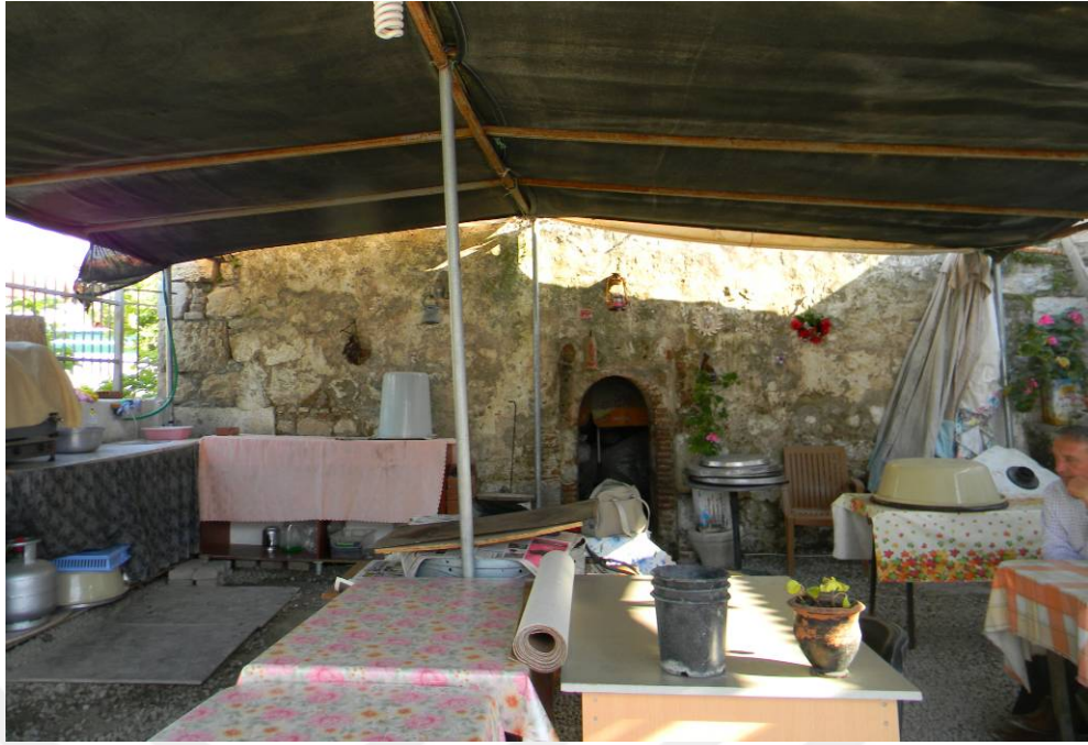
Figure 3.42. Northwest wall of the soyunmalık space.
