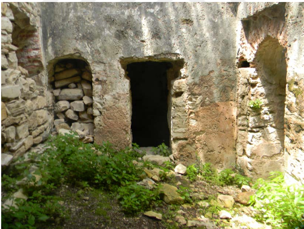
Figure 3.3. Openings on the west wall of the main ılıklik space.
