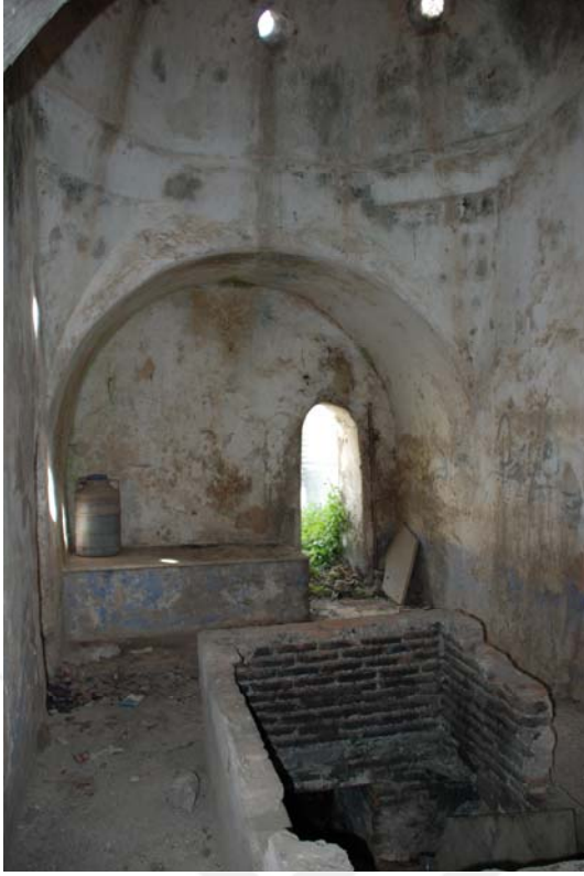
Figure 3.48. Eastern iwan in main sıcaklık .
