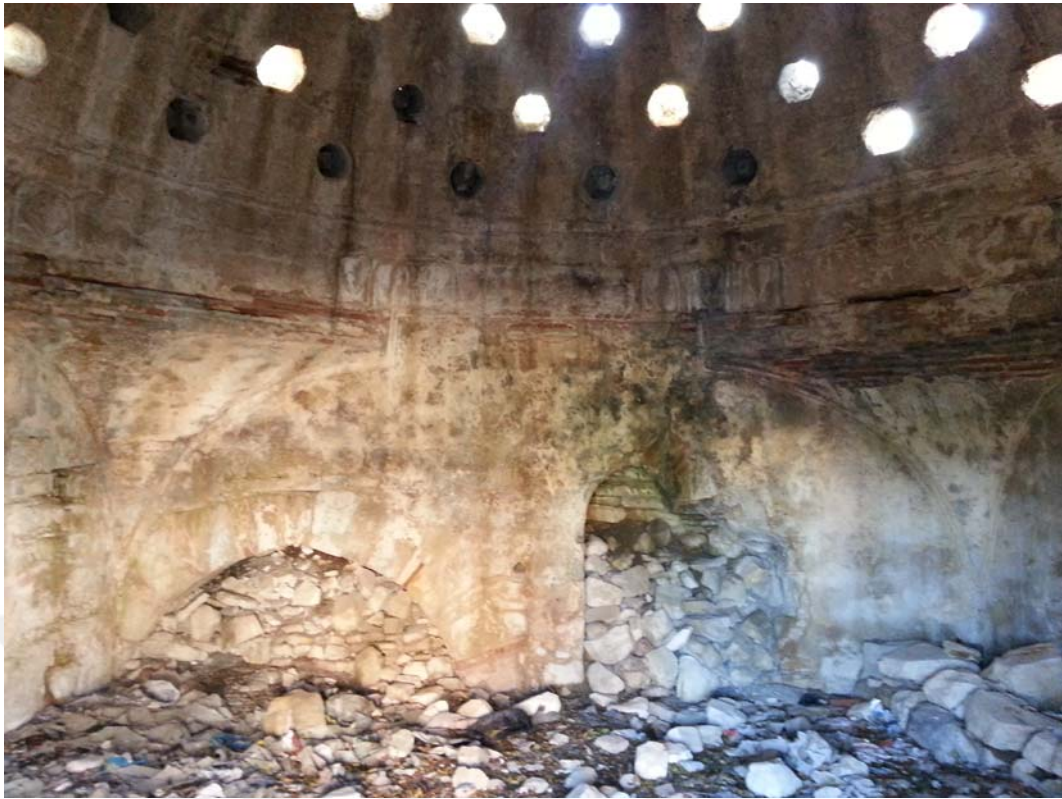
Figure 3.14. Closed openings on the southeast wall of the space.
