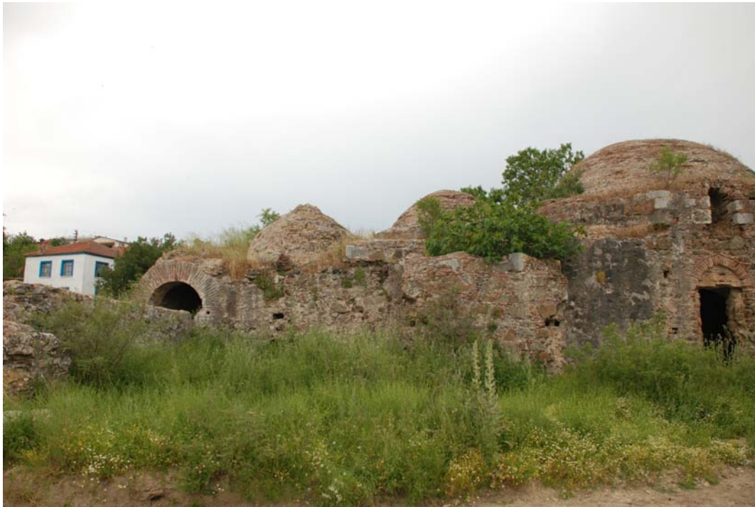
Figure 3.35. General view of the bath from the east.
