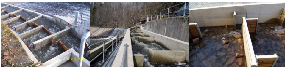
Figure 2.8: Vertical slot fish passage, from left to right: Rochsburg, Poppenwald, Rochlitz (Saxony Dam Administration, 2014).
