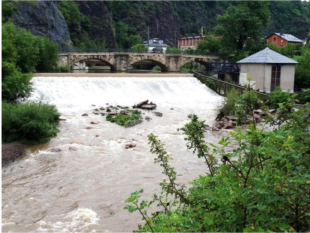
Figure 5.3 : WKA Bienertmühle weir, fish passage and hydro power plant (July, 2014).
