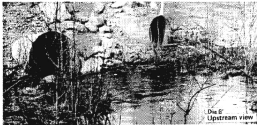
Figure 2.9: Upstream view of roadway culverts in Alaska (Kane and Wellen, 1985).
