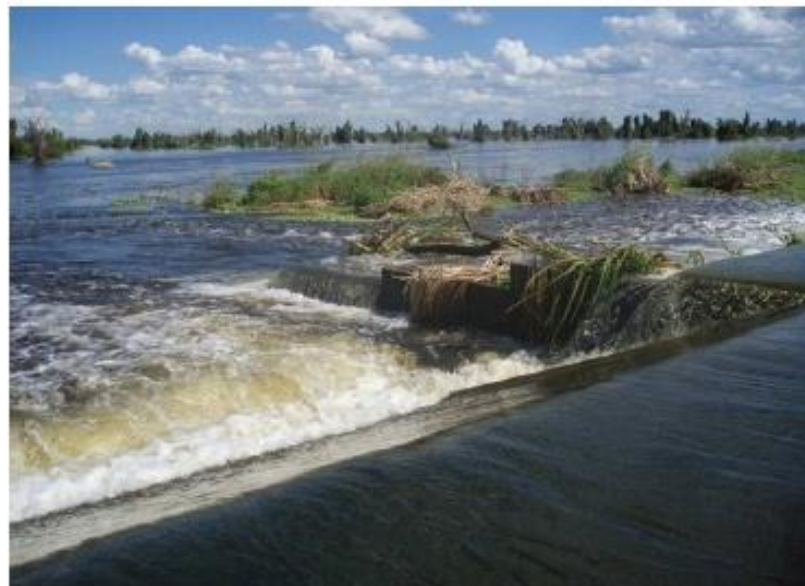
Figure 2.11: View of a fish ladder (pool and weir system) in Rio Paraopeba (Alves, 2007).
