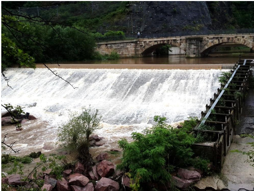
Figure 5.4 : Vertical slot fish passage structure next to WKA Bienertmühle weir (July, 2014).
