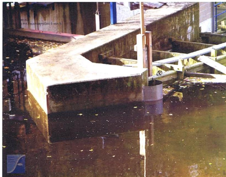
Figure 6.3: Close-up view of fish passage at WKA Bienertmühle weir (2014).
