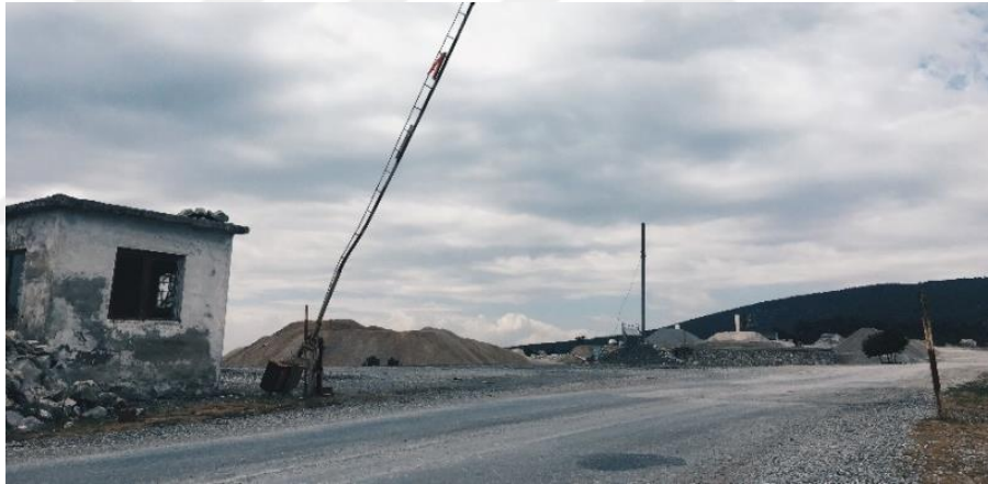
Figure 6.12. Quarry at Kurudere Village, Bornova. 301
