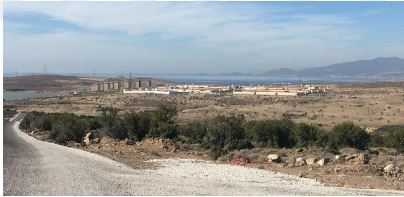
Figure 6.41. Prison at Bahçedere Village, Aliğa. 331
