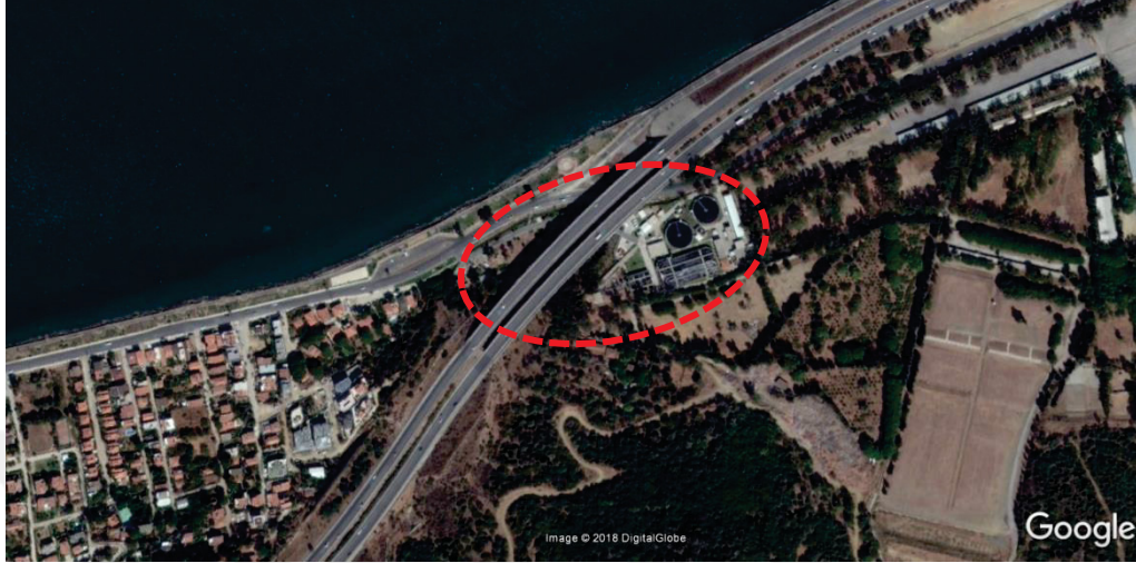
Figure 14. Location of The Southwestern Advanced Biological Wastewater Treatment Plant (Source: Google Earth, 2018)
