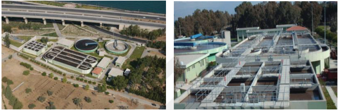
Figure 16. Southwestern Advanced Biological Wastewater Treatment Plant Units (Source: İZSU, 2018)
