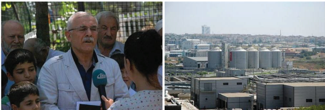
Figure 9. The Ambarlı Advanced Biological Wastewater Treatment Plant in İstanbul (Source: Milliyet, 2016)
