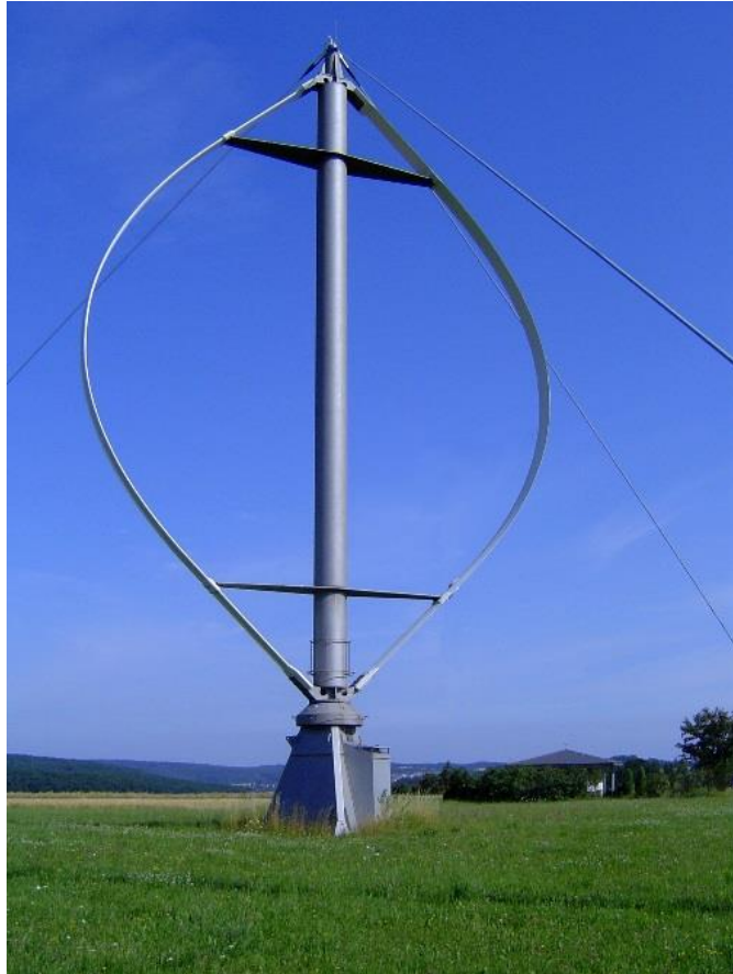
Figure 2.12: Vertical wind turbine[13].
