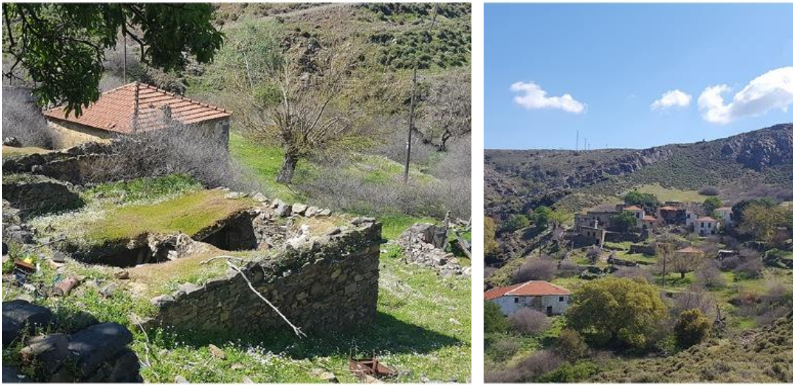
Figure 4. 39. Views of houses in Küçükbahçe.
