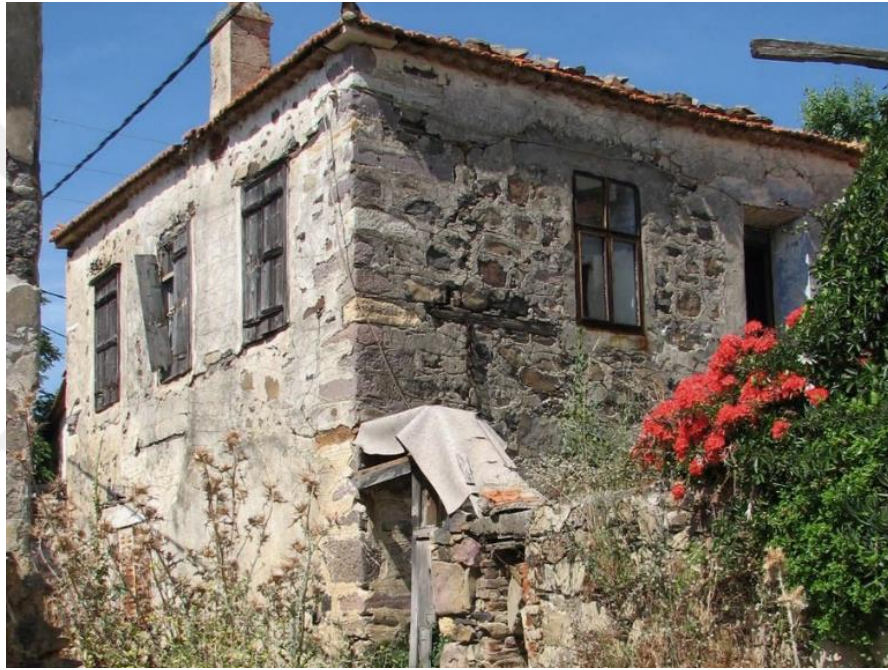
Figure 4. 44. View of stone house. 176
