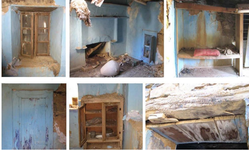
Figure 4. 54. Window, furnace, alcove, meat safe and wooden lintel. 186
