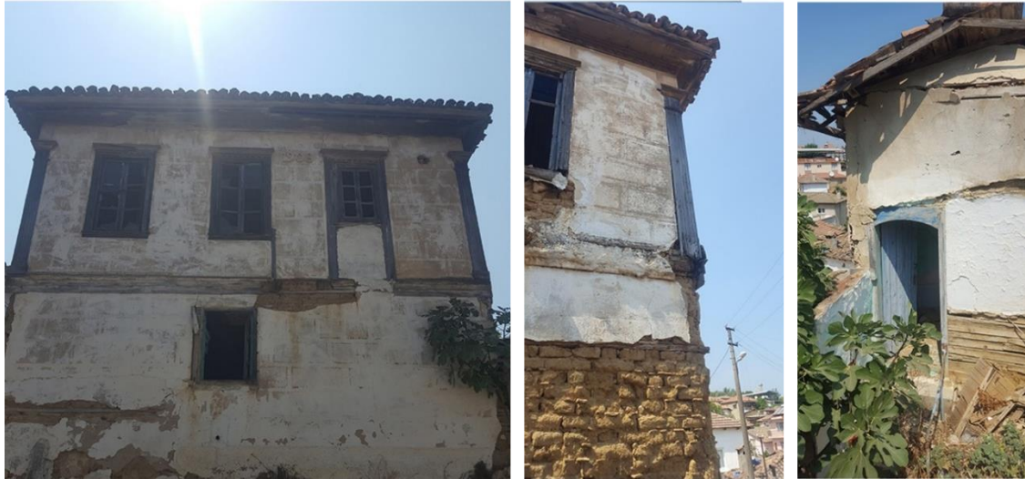
Figure 4. 32. The views of the 1908-built Rum house from different angles.
