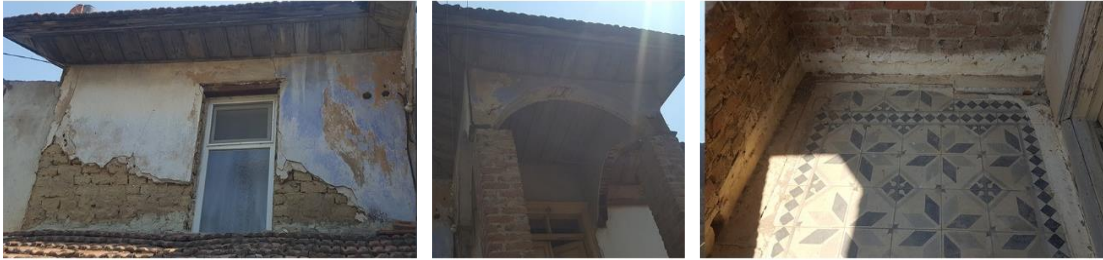
Figure 4. 29. Entrance section with columns made of bricks and patterned floor tiles.
