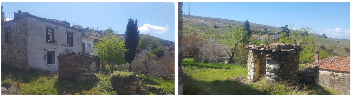
Figure 4. 42. View of a cylindrical toilet that is located outside the house.
