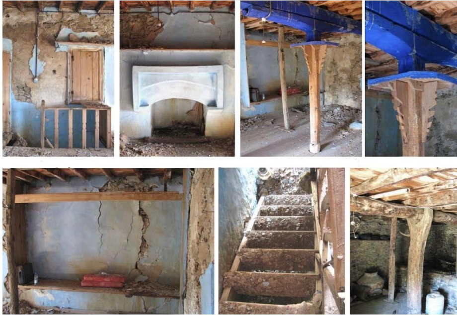
Figure 4. 53. Floor systems carrier beam, stove, and furnace. 185
