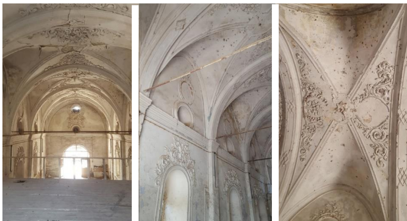
Figure 4. 24. View of vault, covered icons, alcoves and ornaments.
