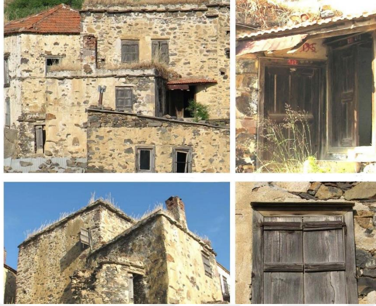
Figure 4. 52. View of stone facade and wood joinery. 184
