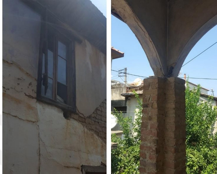
Figure 4. 30. View of a wooden window frame and arch.
