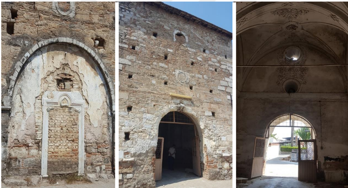
Figure 4. 26. View of doors from inside and outside.
