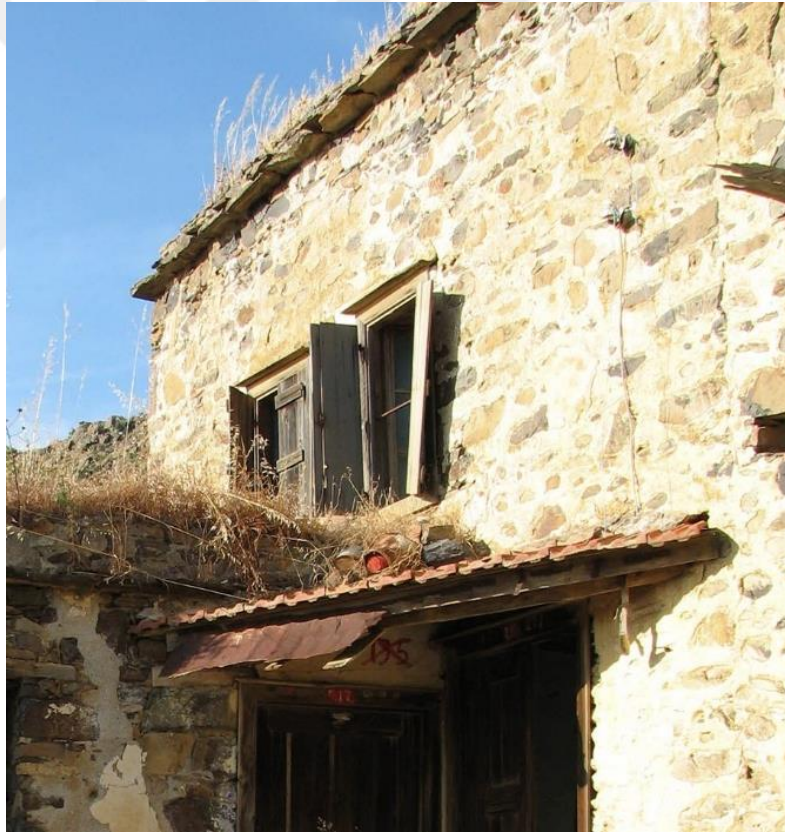
Figure 4. 51. View of two-story house. 183
