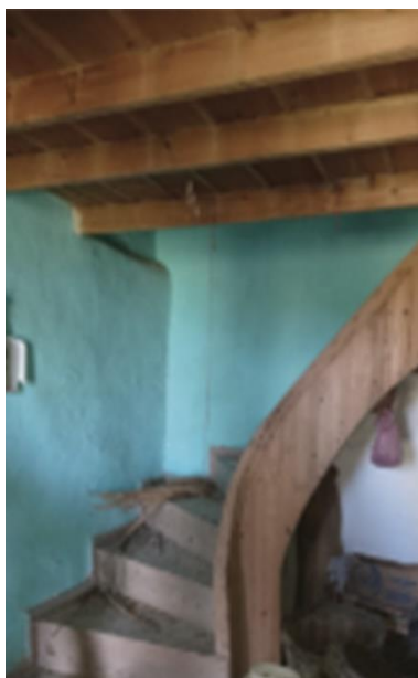
Figure 4. 43. View of inner timber stairs.
