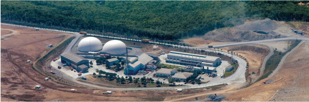
Figure 3.21 : LFGTE plant in Istanbul (Turkish Time, 2011).
