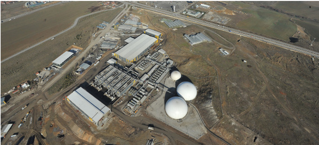
Figure 3.23 : LFGTE plant in Ankara (ITC Turkiye).
