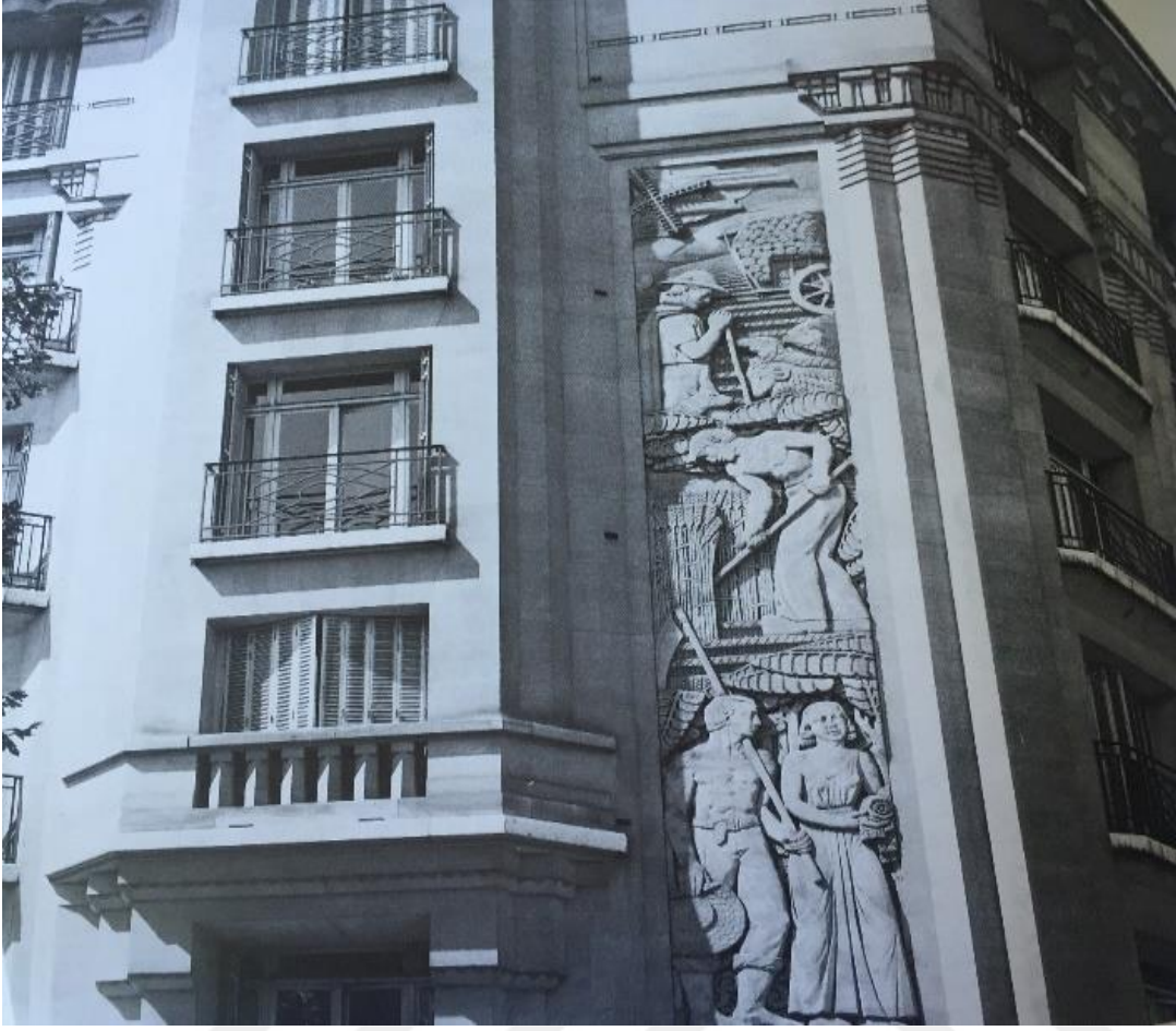
Şekil 3.53: Paris Apartment Building, J.Hilliard, 16 Rue Chardon-Lagache, (Bayer,1992,s.72)
