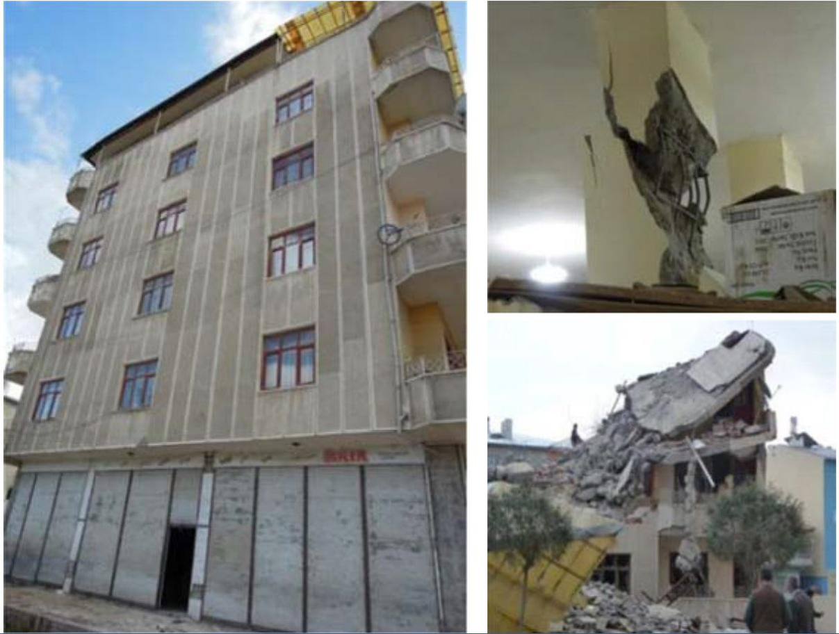
Figure 1.5 After M_w 7.2 heavily damaged, after M 5.6 collapsed [4]
