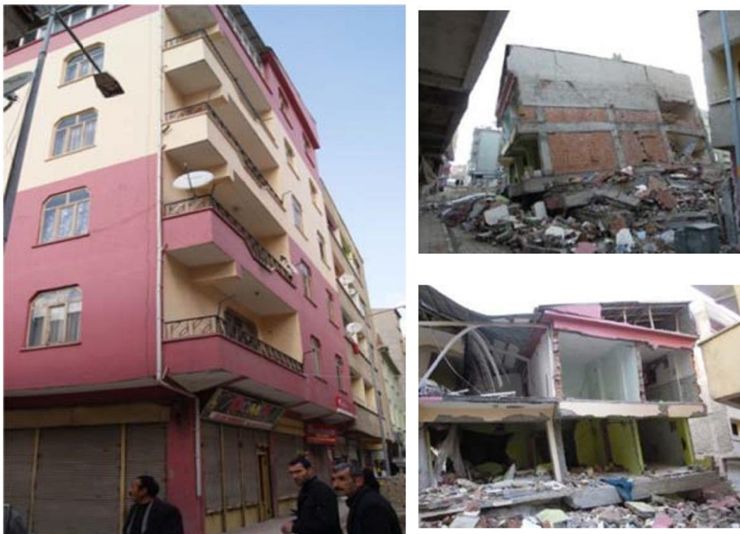
Figure 1.4 After M_w 7.2 heavily damaged, after M 5.6 collapsed [4]
