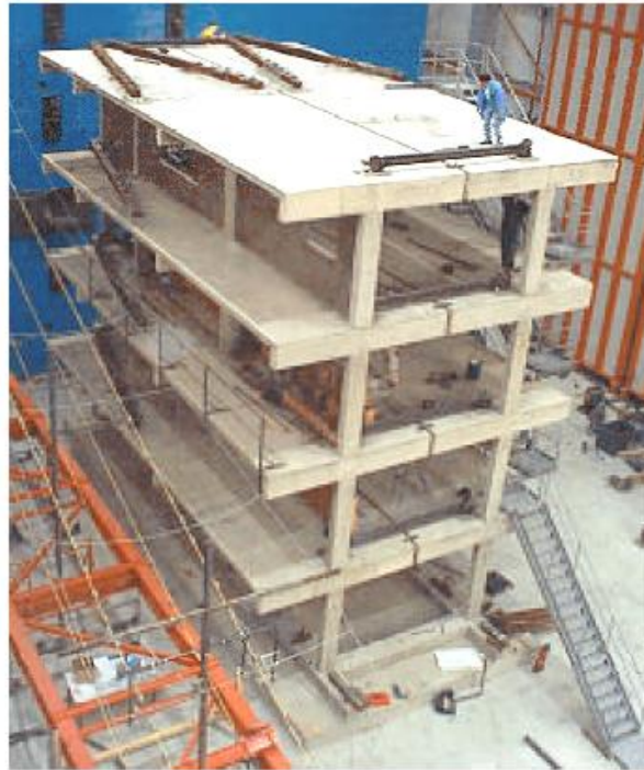
Figure 3.5 : General view of the structure
