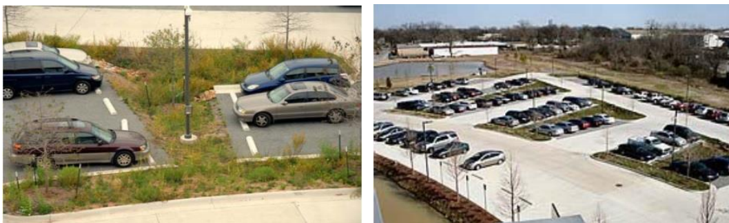
Figure 3.29 : Green parking lot in Heifer International (Letzeiser, 2012).
