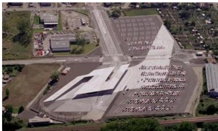
Figure 3.20 : Park and Ride Tram Station (Url-17).
