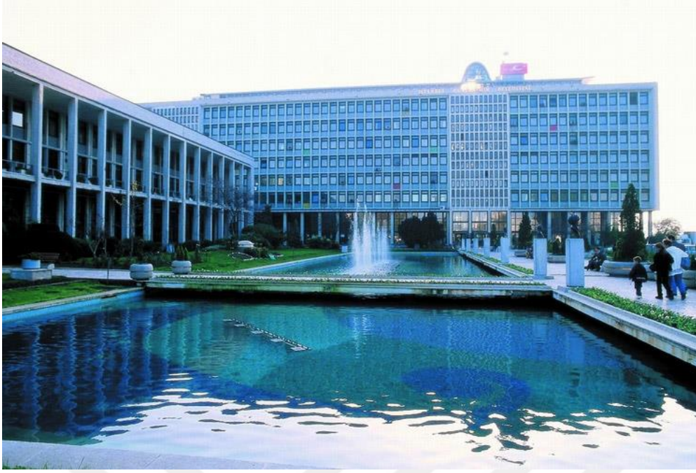
Figure 4.31 : The open plaza and public space of the City Hall (Url-28).
