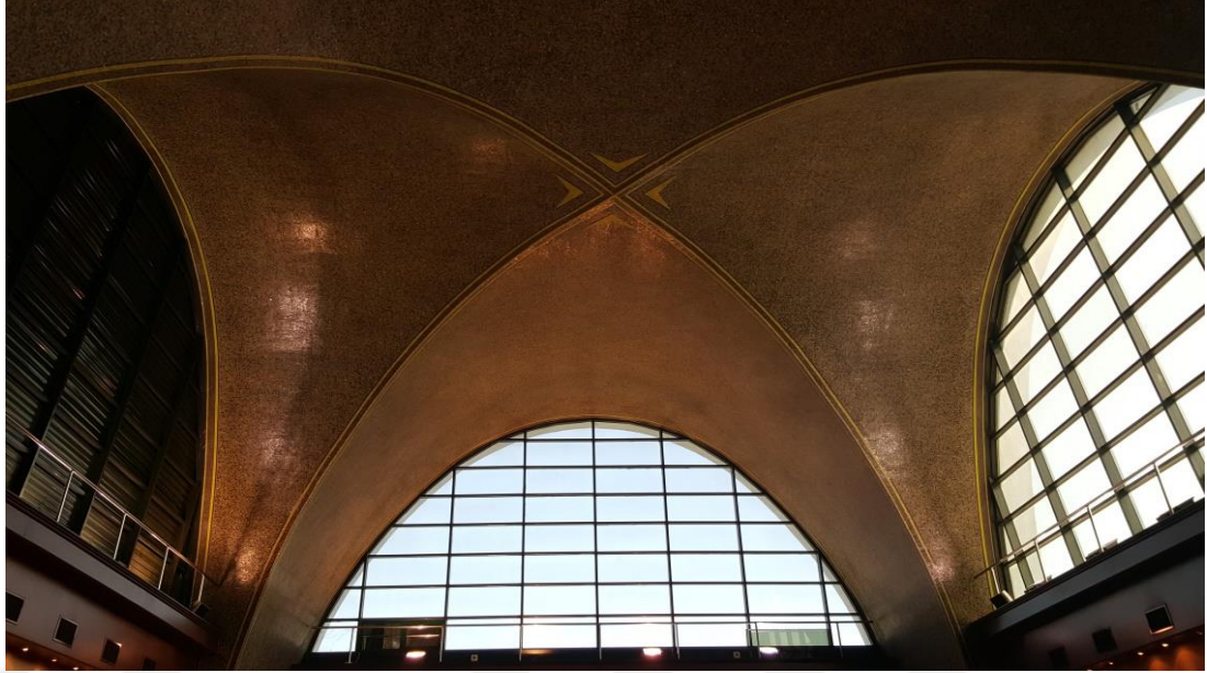
Figure 4.53 : Interior view of the parabolic vault from the of the council chamber (Çetinel, 2015).
