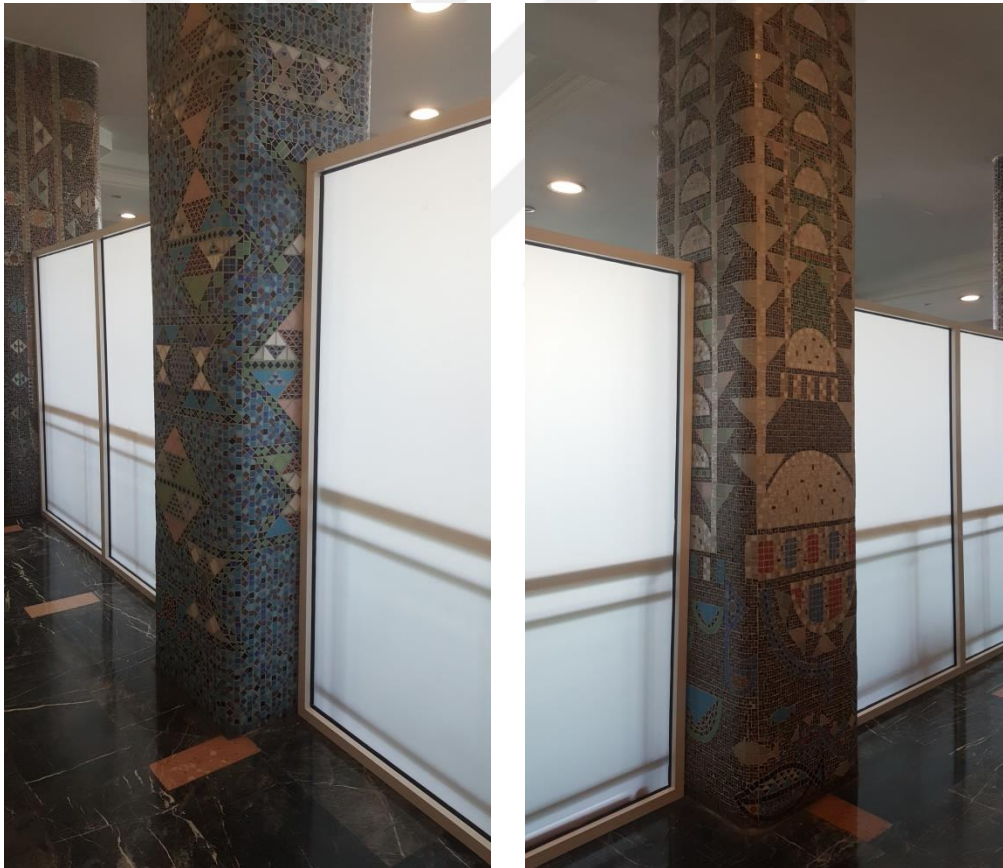
Figure 4.46 : The current view of the mosaic covered columns, separated with elements for new functions (Çetinel, 2017).
