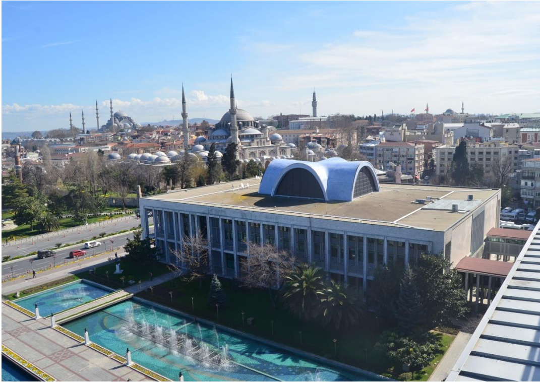
Figure 4.27 : External view of the dome from the roof of the office block (Şevkin, 2015).
