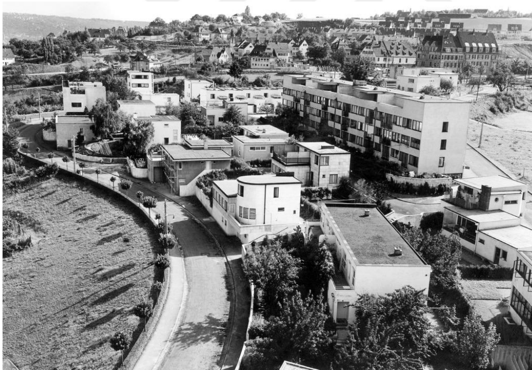
Figure 2.2 : General view of the Weissenhofsiedlung (Url-3).
