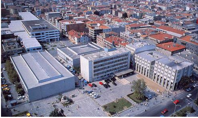
Figure 4.37 : Aerial view of the Sakarya Government Office showing the mass and open area relationship (Url-29).
