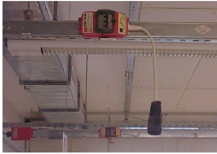
Figure 9: Overhead electric (power) lines and cable trunking systems (photography by the author)
