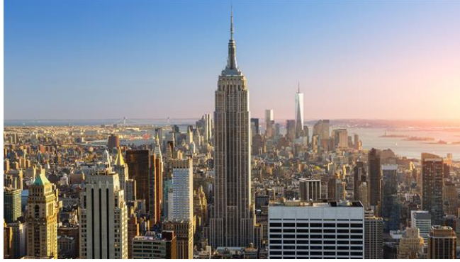
Şekil 2.5: New York Empire State Building.
