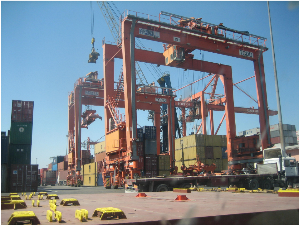
Figure 2-3: Gantry crane in Port of Izmir
