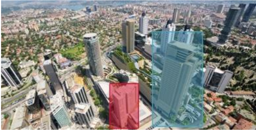
Figure 4.1 : First case study building.
