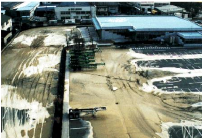
Figure 1.3 : Parking lot on reclaimed land near Ashiya. Sand covering the lot is evidence of large-scale liquefaction and sand ejection (The January 17, 1995 Kobe Earthquake an EQE Summary Report).
