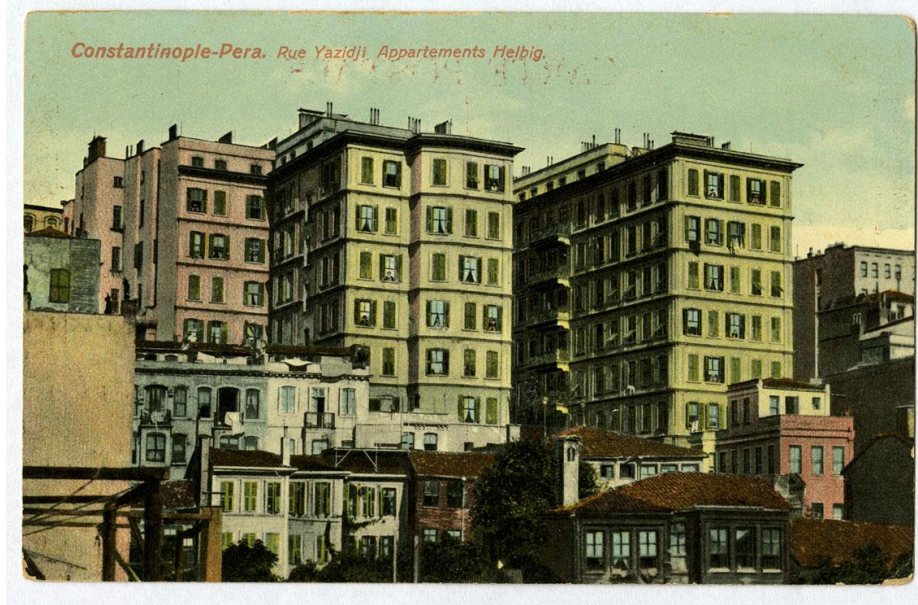
Figure 3. 14: Doğan Apartment Building in Pera, IBB Atatürk Library.
