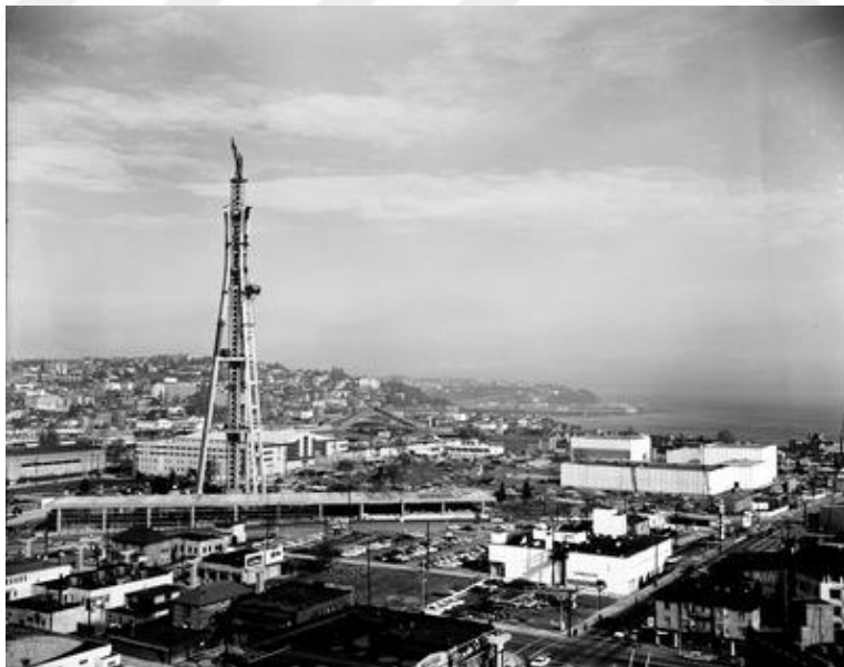
Figure 2. 19: Space Needle for Seattle Fair under construction, Washington, 1962 (URL 21).
