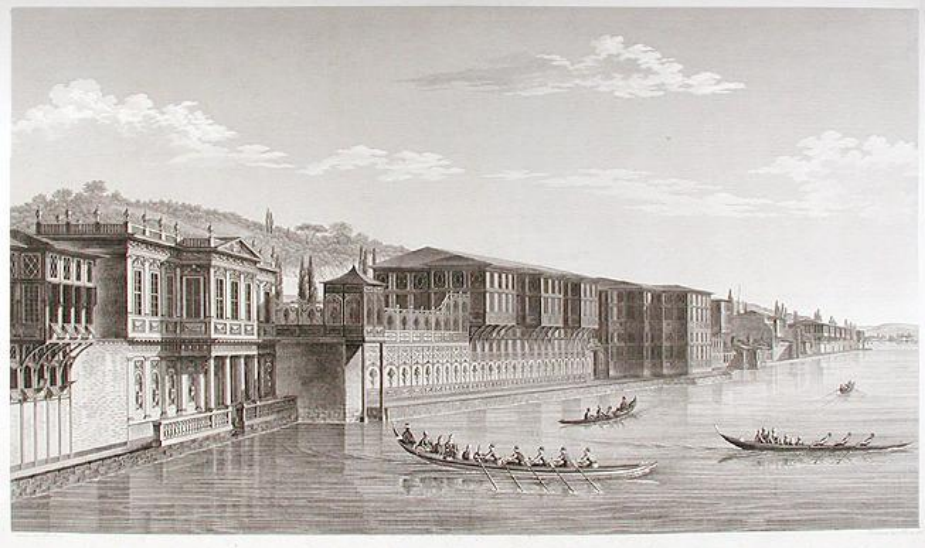
Figure 3. 7: Hatice Sultan Palace in Beşiktaş by A. I. Melling (Melling, 2012).
