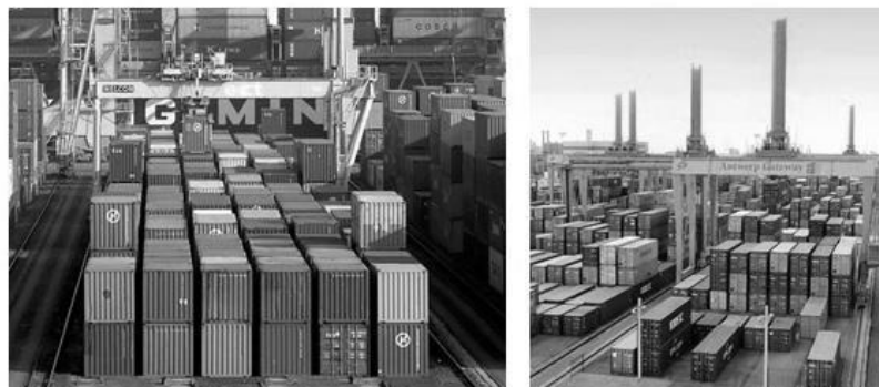
Figure 5 Automated Stacking Crane (ASC)
