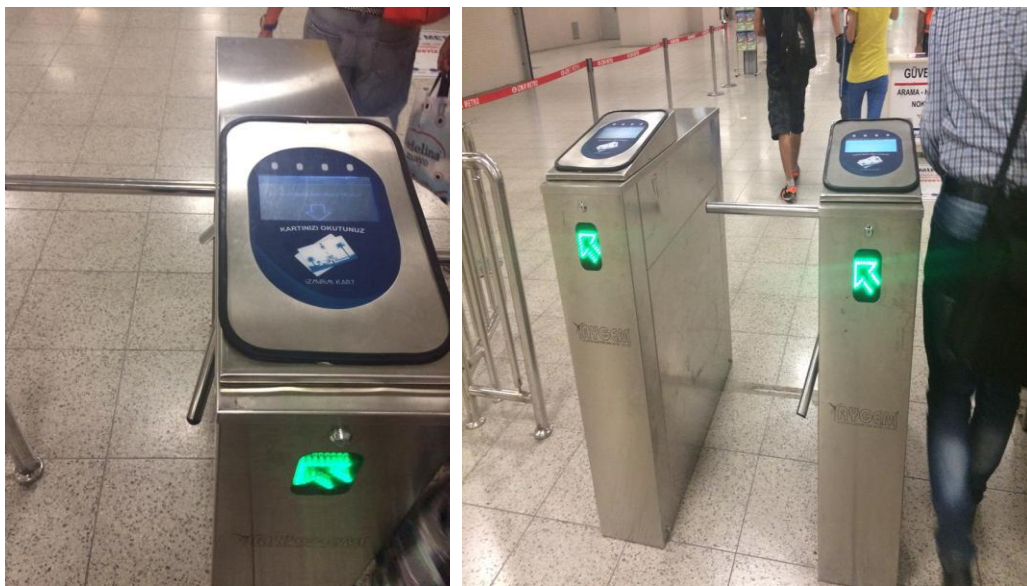
Figure 4 Sensors and turnstiles at Fahrettin Altay station entrance
