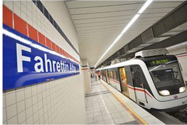
Figure 3 Subway train and station waiting hallway of Fahrettin Altay station
