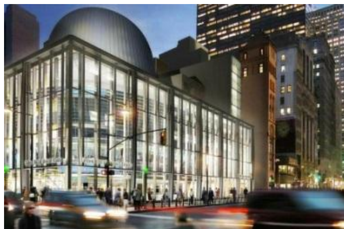
Figure 12 Fulton Station by Grimshaw Architects (Yoneda, 2014).
