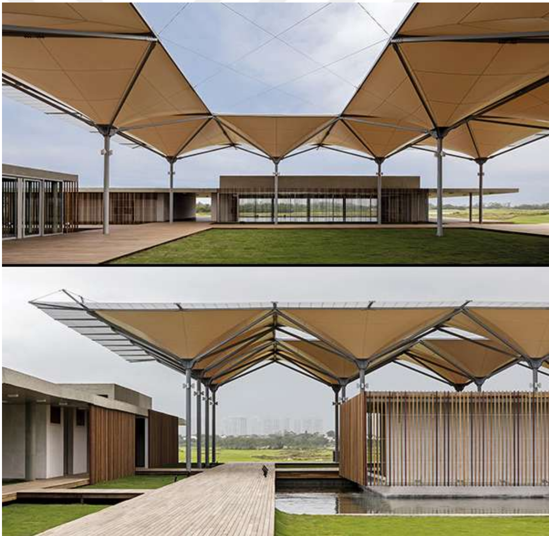
Figure 38 - Olympic Golf Course (Rua Arquitetos: Évora + Rivera) Harvested water is used for irrigation of the golf course.
