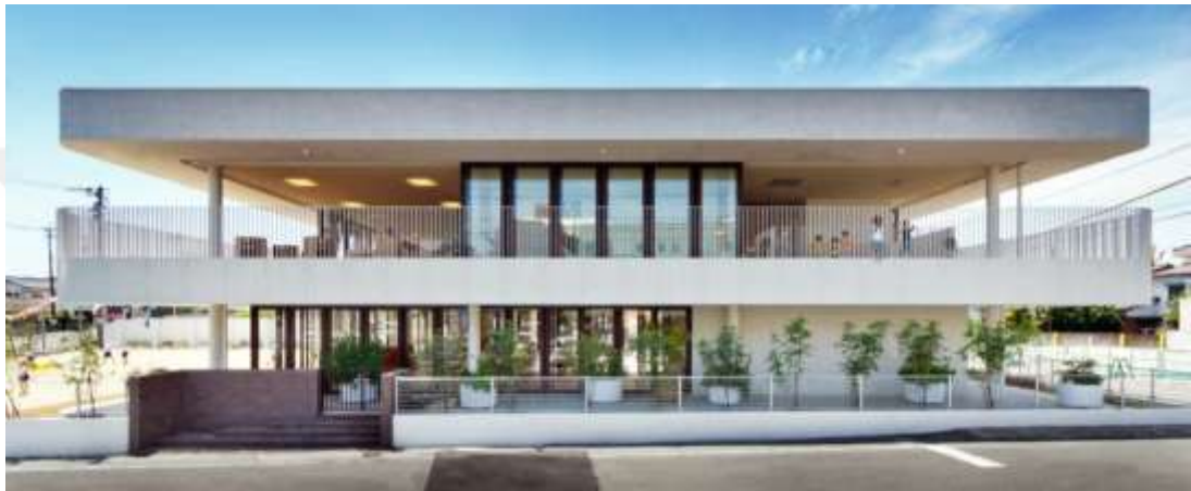
Figure 44 - Front Facade of Dai Ichi Yochien Preschool ( hibinosekkei.com ) The building was designed with plenty of glass walls and natural light for giving flexible and unconstrained qualities to the built space.
