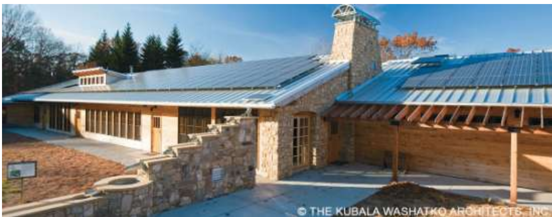
Figure 59 - Aldo Leopold Center (Boldt) In the Kubala Washatko Architects' design for Aldo Leopold Center, conveyance gutters are placed on top of descending separating wall, which also serves as a landscape element.
