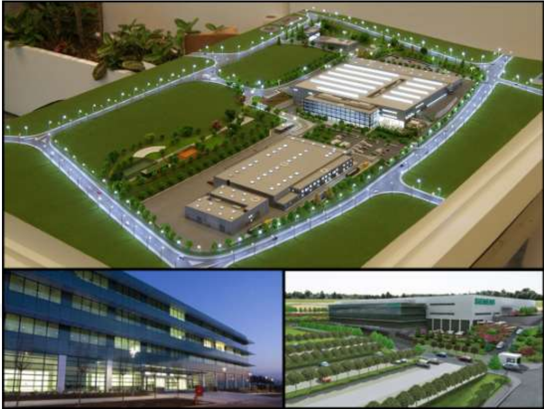
Figure 46 - Siemens Gebze Factory, Kocaeli ( siemens.com; Altın Oran Market ) The photos show a scale model of the site (top), and the entrance of the work space below.
