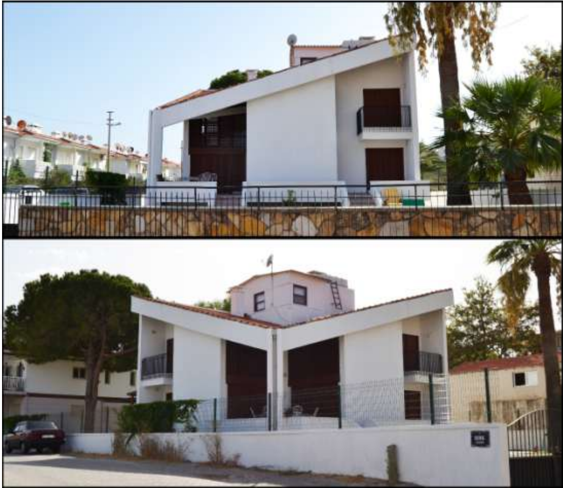
Figure 58 - Ilıca House by Bozkurt & Kavadarlı (photo by the author) Top, the front view of the house; bottom, the corner view.
