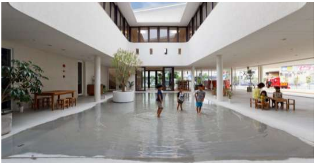
Figure 45 - Courtyard of Dai Ichi Yochien Preschool ( hibinosekkei.com ) The central opening admits rain to the ground floor where the water is retained by the floor shape for children to enjoy playing with mud-free water.
