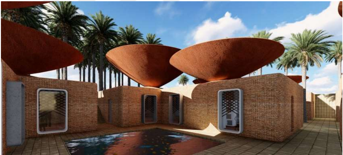
Figure 50 - Primary School Design with Concave Roofs (BMDESIGN Studio, 2017) BMDESIGN's 2017 proposal is come into prominence with its unusual roof design and the importance given to the rainwater harvesting.
