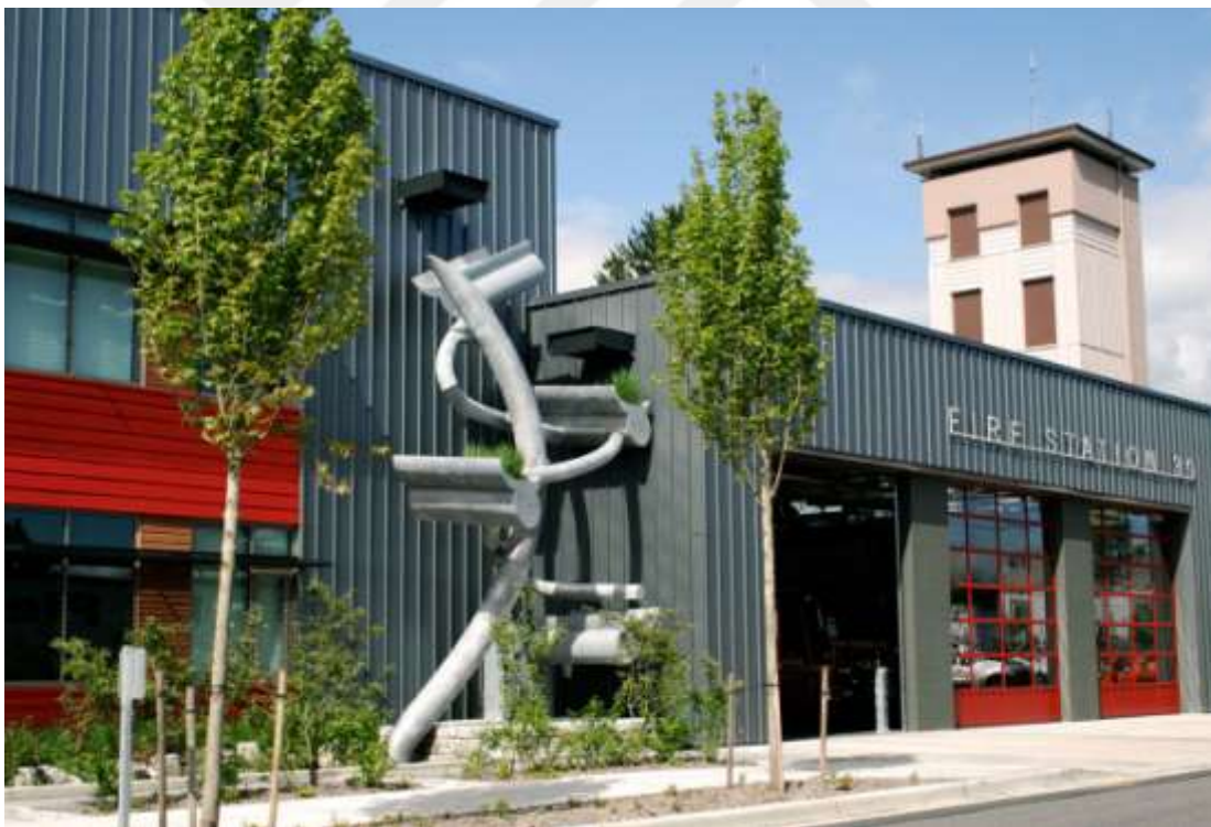
Figure 60 - Stephen Glassman's Thornton Creek ( publicartarchive.org, 2010 ) The free-standing sculpture in the garden of Fire Station 39 in Seattle, Washington, is visually and functionally integrated with the rainwater delivery system, moving runoff from the building's roof to an underground water tank.
