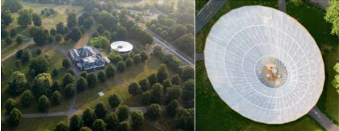
Figure 35- Top View of Serpentine Pavilion of Kéré (Kéré Architecture) At the center of the Pavilion, there is a large opening in the canopy, creating an immediate connection to the sky.
