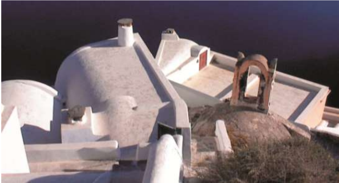
Figure 49 - Back View of the Altered Roof from Santorini
