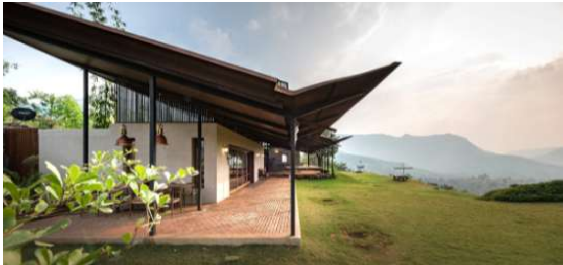
Figure 55 - Side View of the Y-Shaped Roof ( spasmindia.com )
