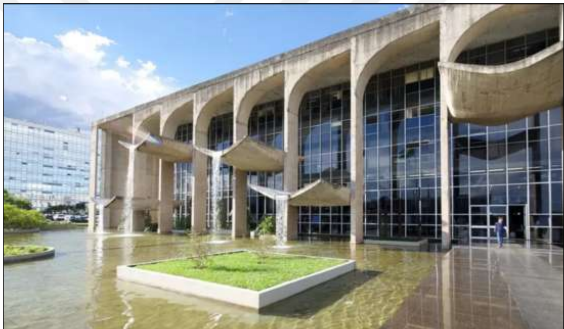
Figure 57 - Waterfall on a Facade of Justice Palace in Brasilia ( expedia.com ) The building is designed by Oscar Niemeyer in 1962 as headquarter to Ministry of Justice and opened in 1972. The square volume sitting on a reflective pool, reinforced concrete structure, arches and pillars on facades are the main characteristics of the building. (Ferreira and Maximo, 2013)
