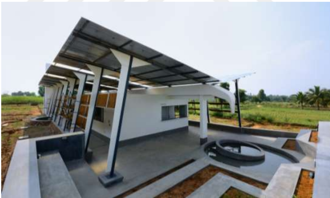
Figure 43 - Rainwater Pond of Dharmapuri Primary Healthcare Center
