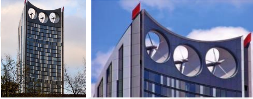
Şekil 3.14 : Strata Tower, WS Atkins & Partners, BFSL, London, 2010 (Url-12).
