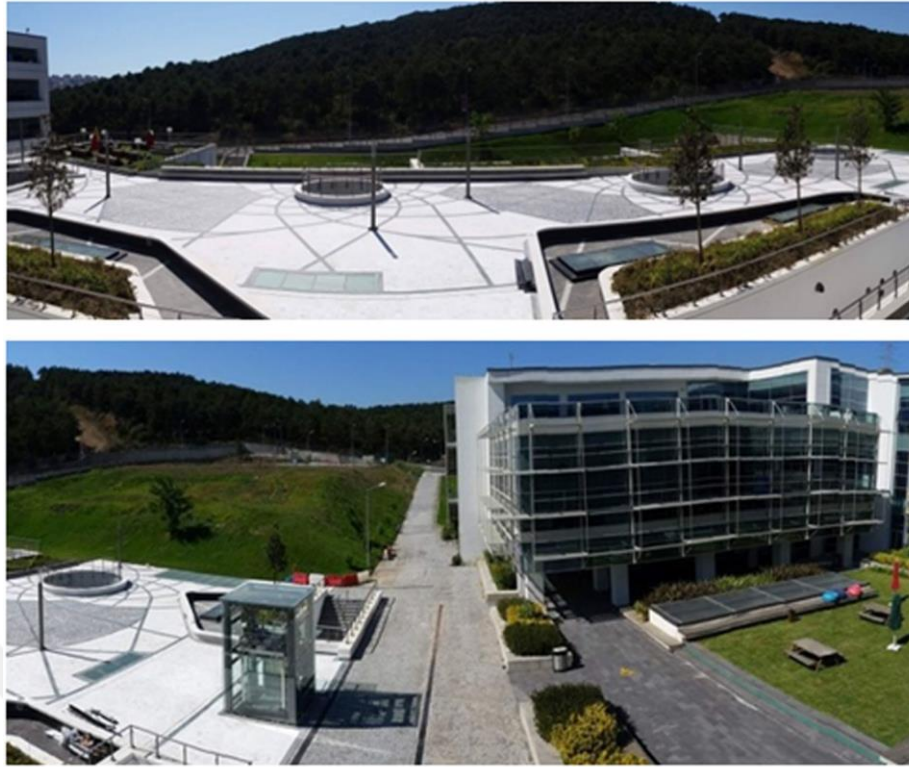
Figure 3.13: View of the pilot study area.
