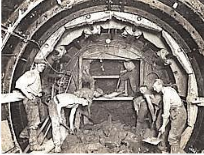
Şekil 2.11: The Greathead Shield (Carrol, 2005).
