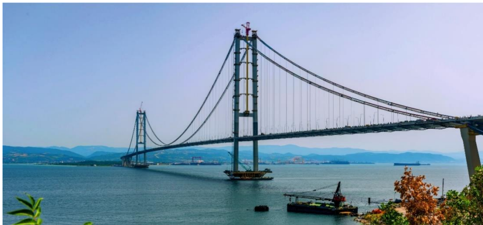
Figure 1.11 : Osman Gazi Bridge
