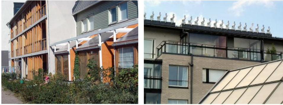
Figure 3.11 : Buildings with solar systems in Eko-Viikki (Hakaste et al., 2005).
