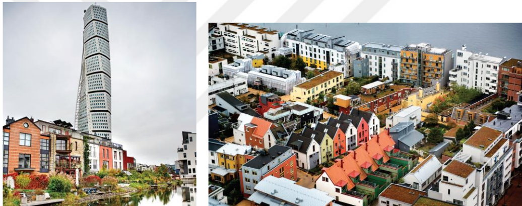
Figure 3.8 : Low-rise buildings in the inner part in Bo01 (Anderberg, 2015).
