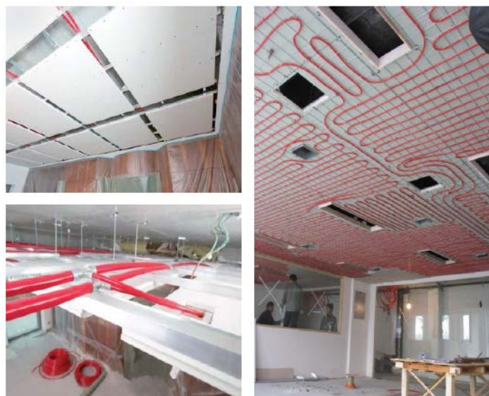
Figure 5.7 : The image of chilled ceiling system application.
