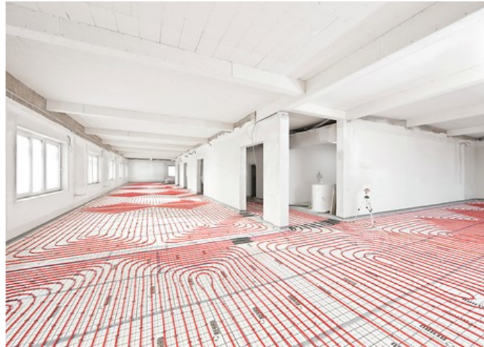
Figure 5.6 : The image of radiant heating system application.
