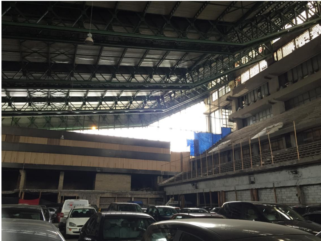
Figure 4.3: Boro-Ramiz Complex. View from The Universal Hall. Beam-Truss System Used for Covering Huge Areas, (Sylejmani, 2017).
