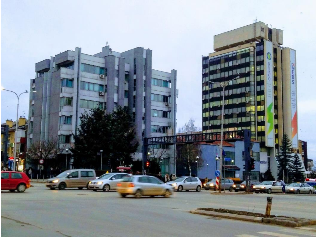
Figure 3.20: Postmodern building in Prishtina. ' KEK Building ' by Zoran Zakic, (Investbiro) in 1984 (Sylejmani, 2019).
