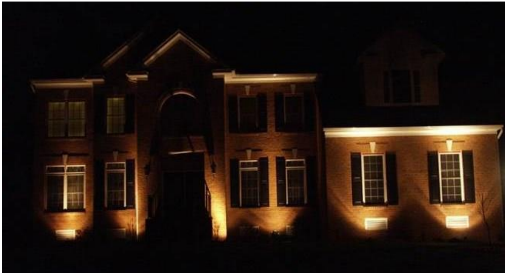
Figure 3.5: Example application of lighting mistakes- Bad fixture placement (Bui,2005).
