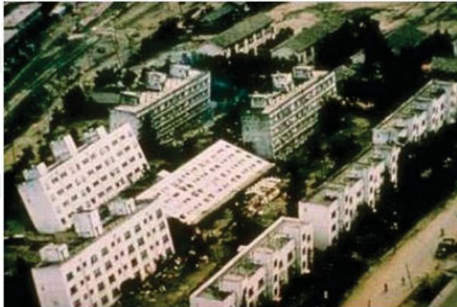
Figure 3.1 : Liquefaction at Niigata earthquakes in 1964 (kramer,1996).
