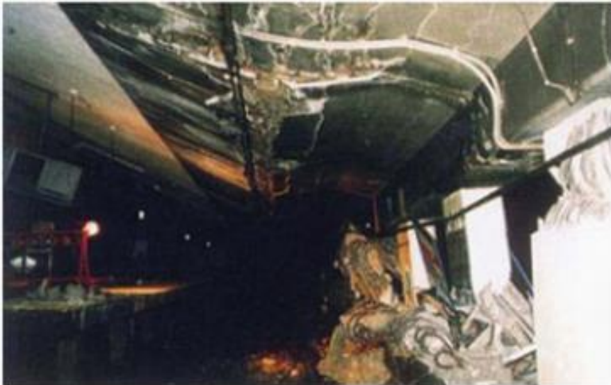
Figure 1.1 : Daikai subway station. (a) Settlements of the overlaying roadway caused by the subway collapse. (b) Collapse of the central columns of the station.
