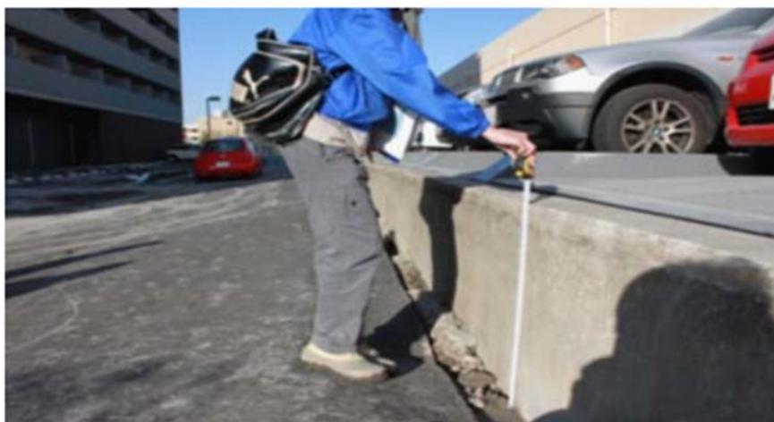
Figure 2.2 : Uplift of parking lot during Tohoku Pacific Earthquake 2011 (Tokimatsu et al, 2012).
