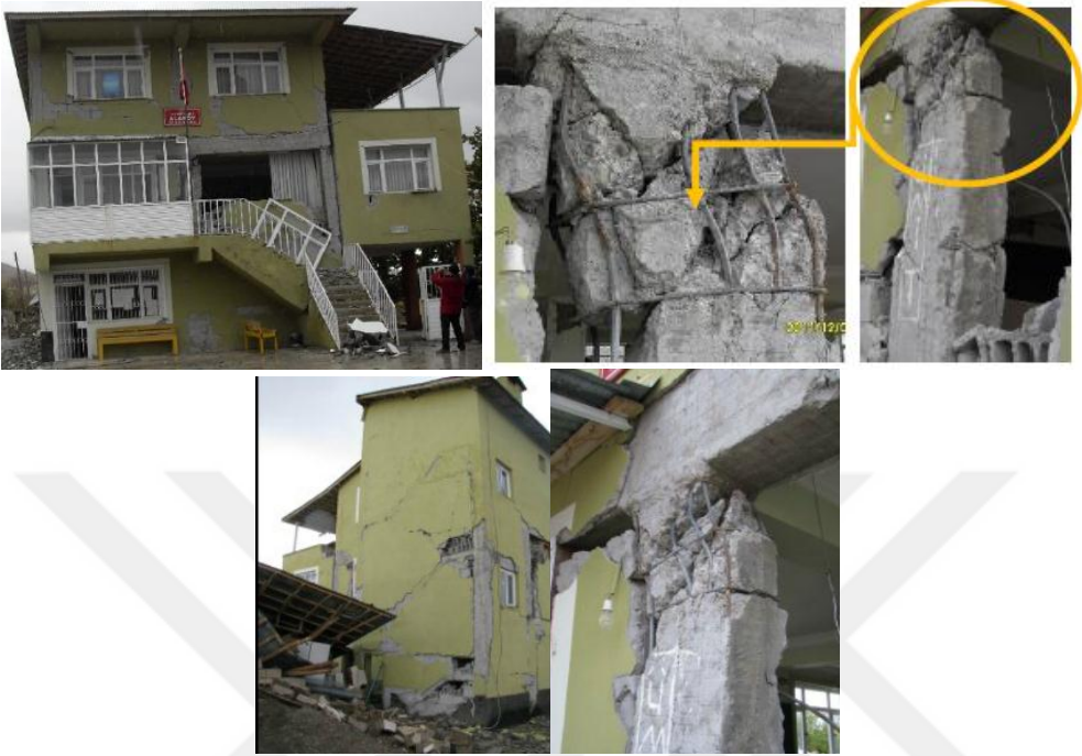
Figure 5.11: Photos of Alaköy building from site investigation (Taşkın et. al, 2014; EEDMI, 2011)
