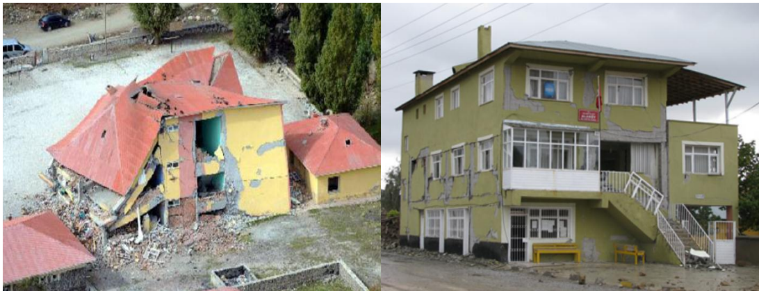
Figure 5.4: Gedikbulak and Alaköy school buildings (EEDMI, 2011).
