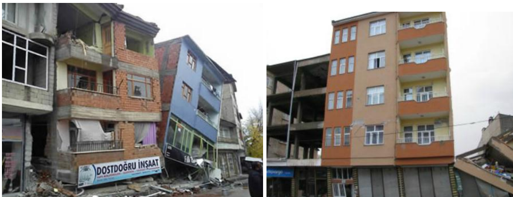
Figure 1.3 : Soft story situation and inadequate separation between adjacent buildings in Van Province (EEDMI Reconnaissance Photos, 2011)
