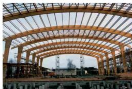
Figure 2.30: Curved rafter portal frame [62].
