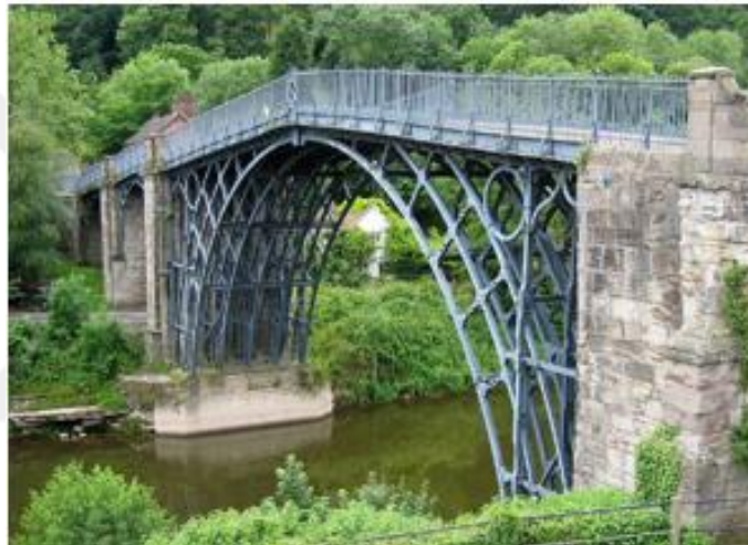
Figure 2.1: Crossing the river Severn, Coalbrookdale, Ironbridge town, Shropshire County, England [9].
