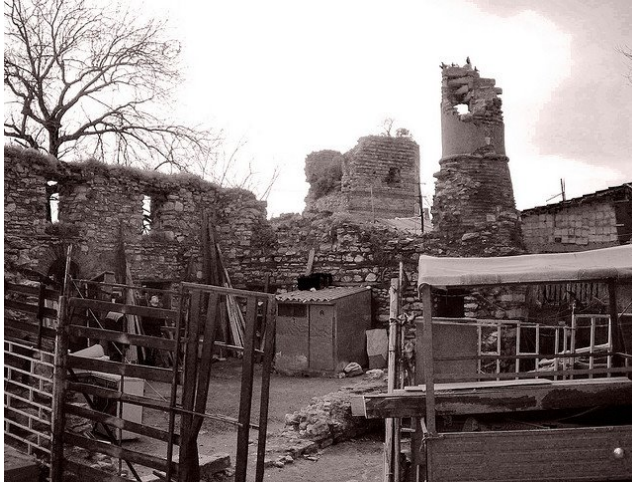
Figure 7.2 The Barn Inside the Tarsus Mosque (Nedim Altınbüken Archive)
