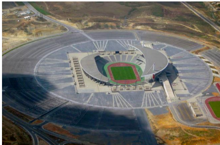
Figure 1.9. Ataturk Olympic Stadium in Istanbul (2005), Original source unknown. Source: http://mapio.net/pic/p-2870209 , accessed December 03, 2017
