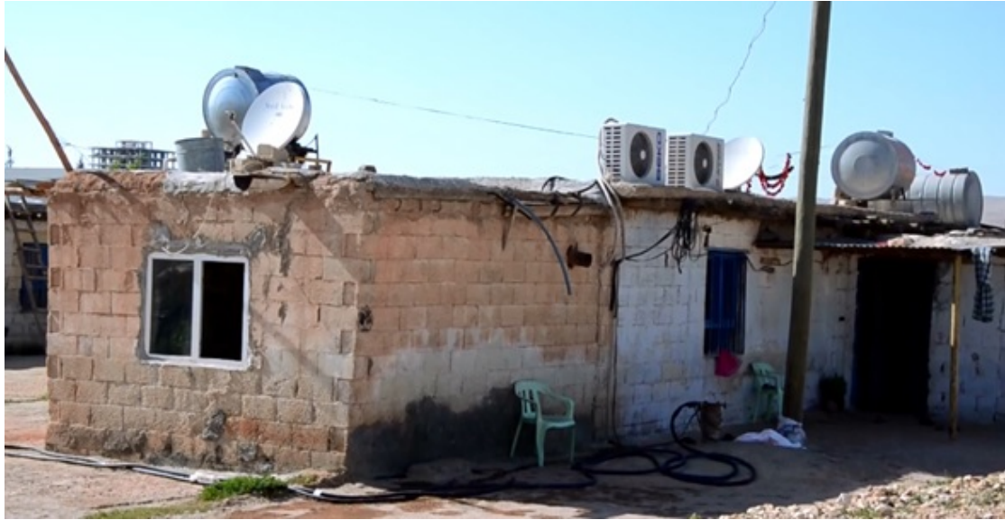
Figure 3.2: A House in the Village with 2 Air Conditioners
