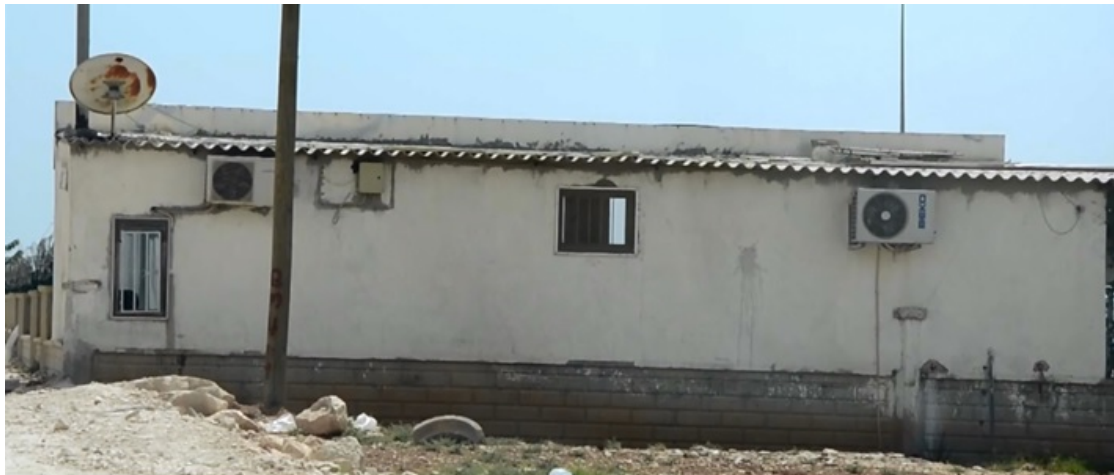
Figure 3.3: A House in the Village with 2 Air Conditioners
