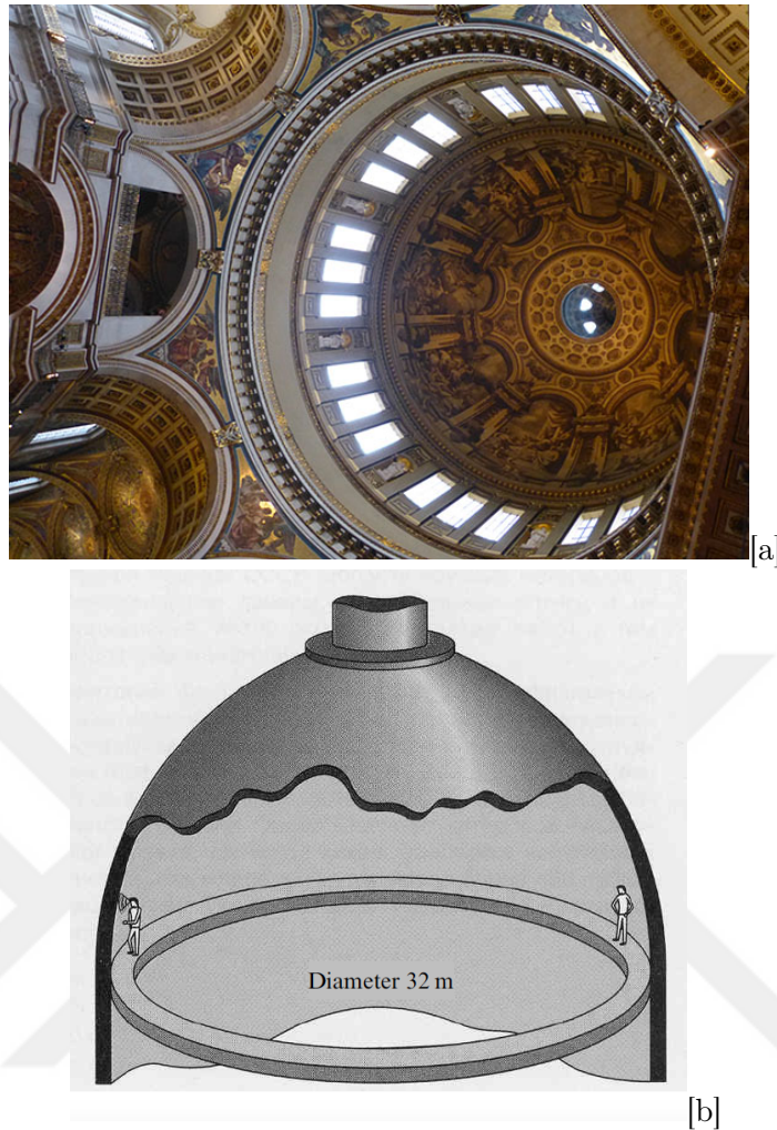
FIGURE 2.9: A picture from the inside view of the dome of the Saint Paul's Cathedral, and a schematic representation of whispering gallery for that dome [21].
