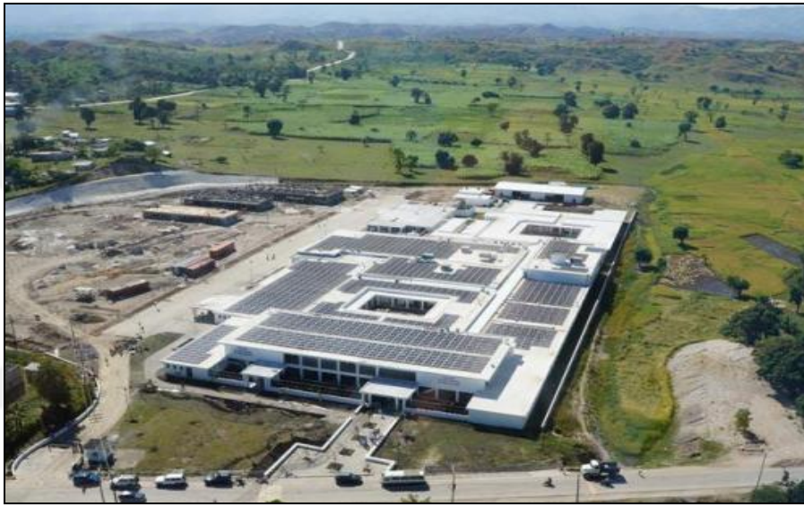
Şekil 3.15 Hôpital Universitaire De Mirebalais Hastanesi Teras Çatı BIPV Uygulaması( http://inhabitat.com/hopital-universitaire-de-mirebalais-will-be-the-worlds-largest-solarpowered-hospital/haiti-solar-powered-hospital-01/ )
