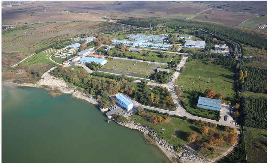
Şekil 4.1 Büyükçekmece İçmesuyu Arıtma Tesisi( https://www.google.com.tr/search?q=b%C3%BCy%C3%BCk%C3%A7ekmece+i%C3%A7me+suyu+ar%C4%B1tma+tesisleri&source=lnms&tbm=isch&sa=X&ved=0ahUKEwj74v-r0jWAhViJsAKHbo2Az8Q_AUICygC&biw=1920&bih=925#imgrc=ZE1XwFqfv4fXIM: )
