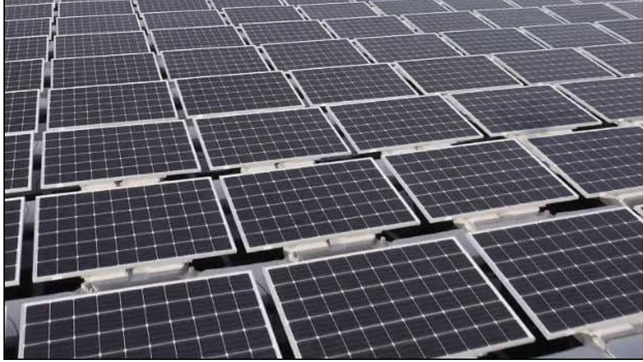
Şekil 3.23 Queen Elizabeth II Rezervuarı Panel Dizilimleri( http://www.telegraph.co.uk/news/earth/energy/renewableenergy/12200484/Europes-largest-floating-solar-farm-powers-up.html ).
