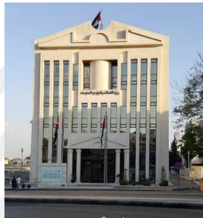
Figure 37 The elevation (Google)
