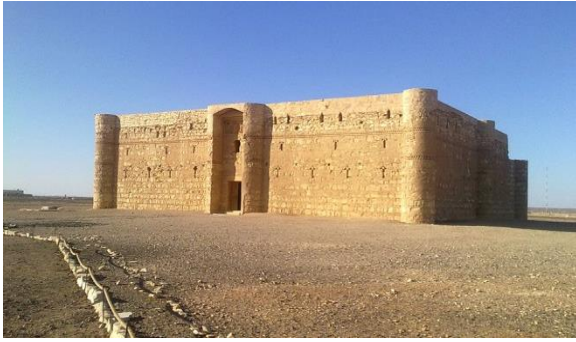
Figure 28 exterior of Qasr, Kharana (Wikimedia, n.d.)
