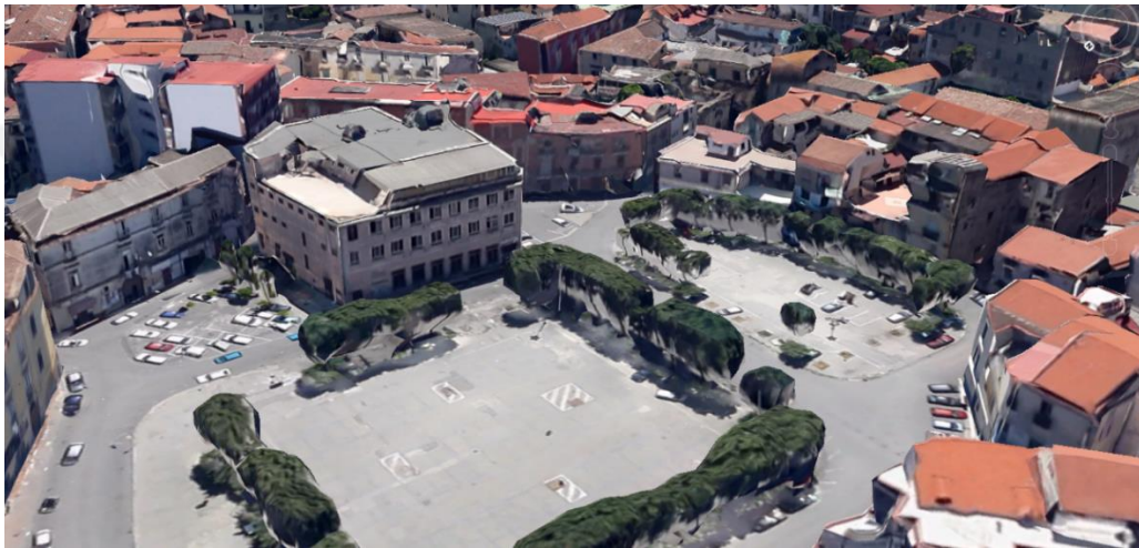
Figure 40. Piazza Marconi- Piazza Marconi-Current situation of C side
