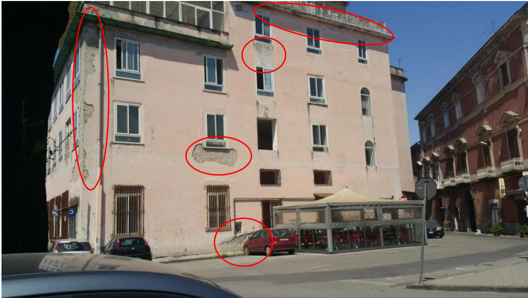
Figure 30.1. 0.5-1,5 cm Plaster Deformations and affusion. (Demirci, Didem,12.06.2017)
