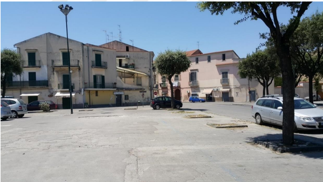
Figure 27.2. Floor Deterioration-3 / Modified Asphalt Operation. (Demirci, Didem,12.06.2017)
