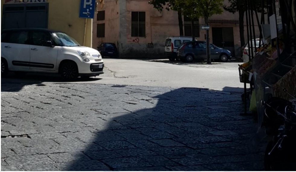
Figure 29.2. Asphalt Deterioration-2 / Multilevel Asphalt Degradation.
