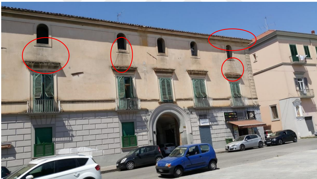
Figure 30.2. Facade Corruption depend on Squalidity and 0.5-1,5 cm Plaster Deformations and affusion. (Demirci, Didem,12.06.2017)
