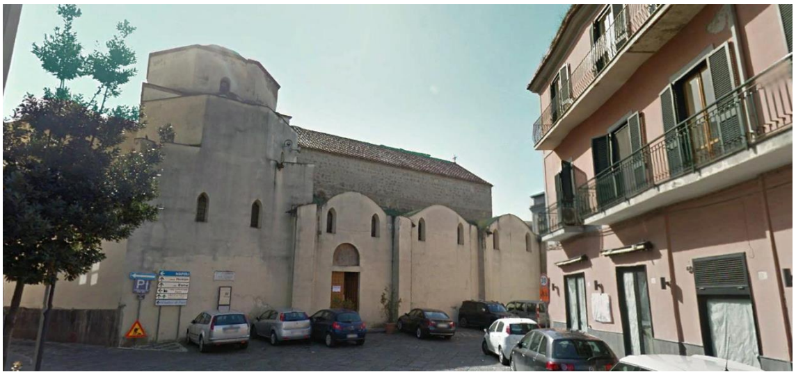
Figure 18.2.North Side Facade of Church of Santa Maria in Piazza (Demirci, Didem,12.06.2017)
