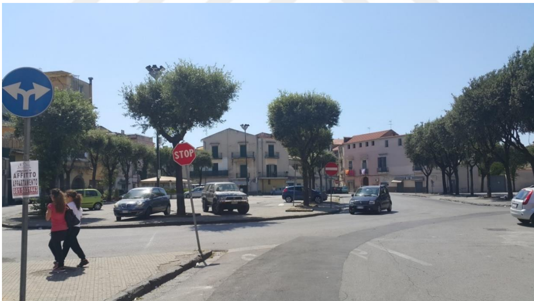
Figure 29.1. Asphalt Deterioration-1/ Patch Operation
