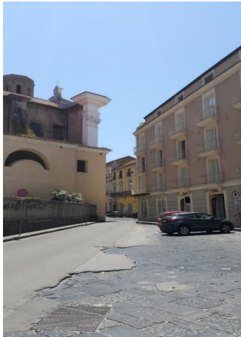
Figure 29.3 Asphalt Deterioration-3 / Asphalt Application on Granite & Multilevel Asphalt Degradation. (Demirci, Didem,12.06.2017)
