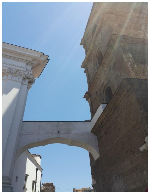
Figure 17.3. Fasade of Cathedral of St. Paul (Demirci, Didem,12.06.2017)
