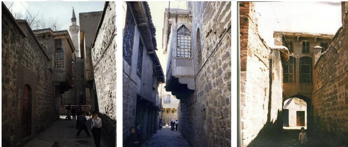
Figure II.11. House Façades and narrow streets in the old town of Diyarbakir (Baran, M., Yıldırım M., Yılmaz, A.2010)
