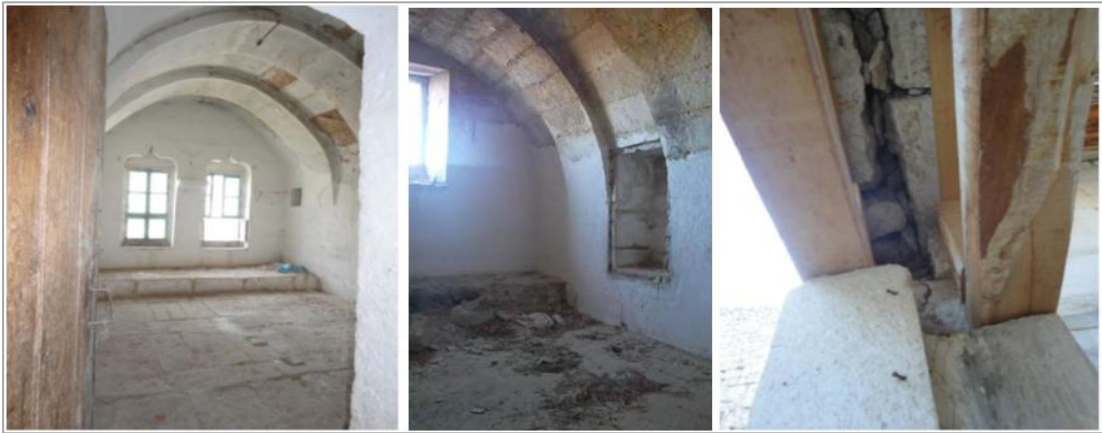
Figure II.14. The thickness of Inner faces of the wall stones, Ürgüp increases time lag( Solmaz, F., Şakar, N. Güçhan, Ş.,2012)
