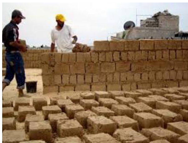
Figure 2.4 Showing to build walls (Abdelslam, 2017)
