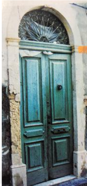
Figure 7.58 The form of Third Entrance of the Housh
