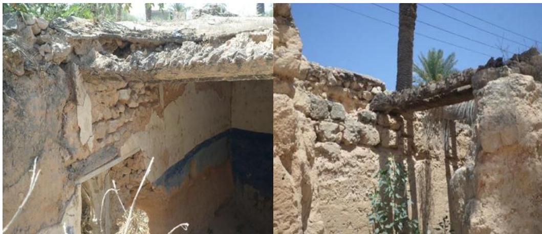
Figure A2.3 The form of ceiling with palm trees Illustrates internal materials (Adeema, 2015)
