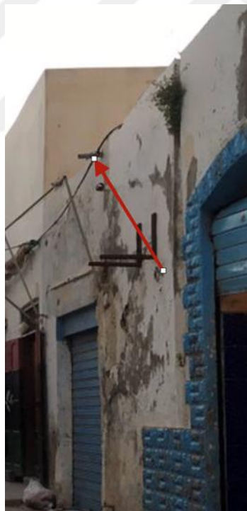
Figure A2.7 The form of The Mizab (waterspout)
