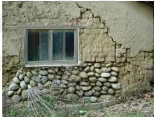
Figure 2.3 Showing the wall (Abdelslam, 2017)
