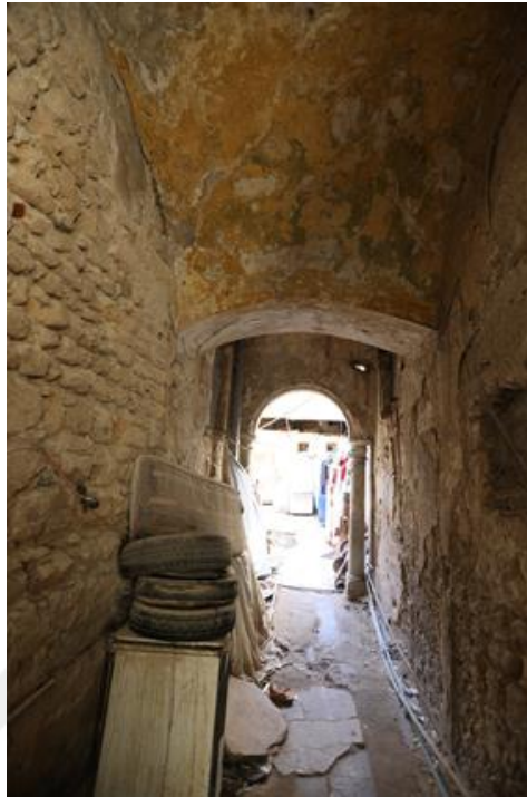
Figure 7.77 Images of the Entrance from the inside of Housh AL-Qurji
