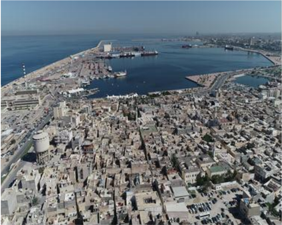
Figure 3.19 An aerial view of the old city of Tripoli
