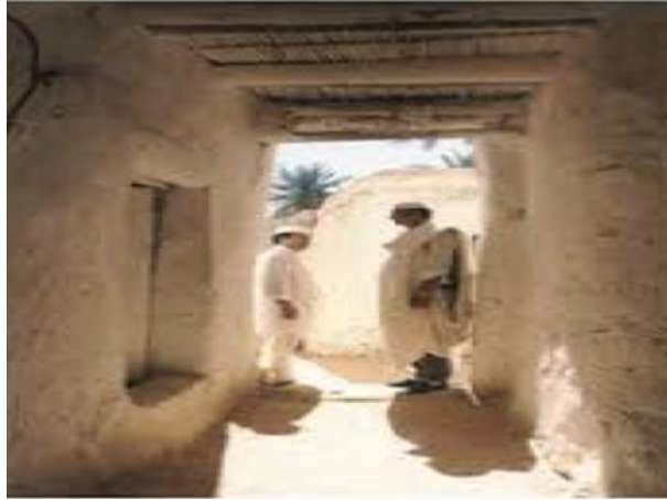
Figure 2.5 Use Palm trunks in ceiling (Abdelislam, 2017)
