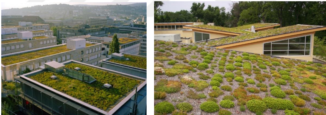
Figure 3.18 Extensive green roof applications [URL24,25]
