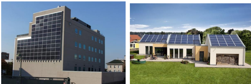
Figure 3.37. The use of photovoltaic panels in buildings [URL39,40]
