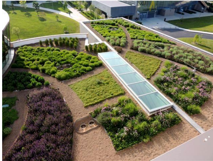
Figure 3.25 Semi-intensive green roof [URL29]
