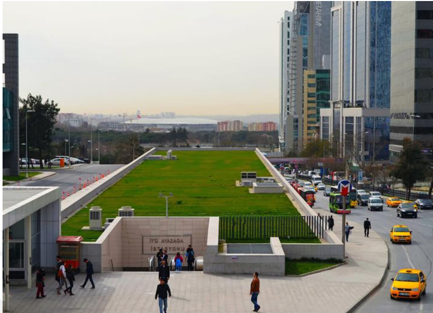
Figure 3.20. Extensive green roof - ITU Ayazağa metro station [URL27]
