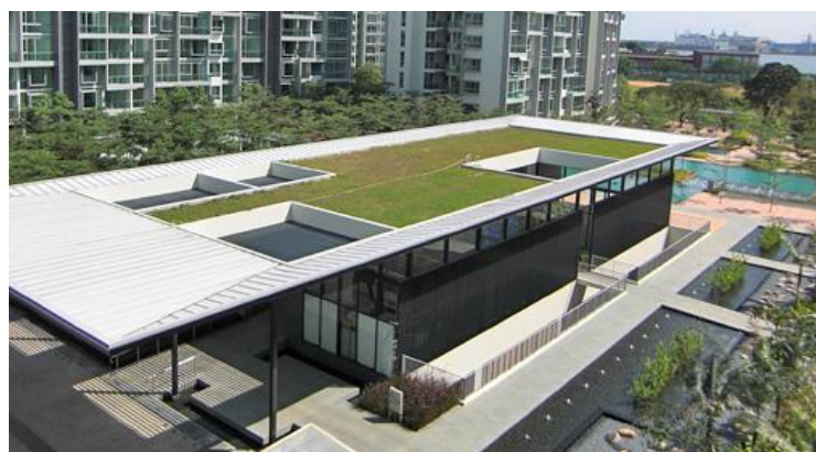
Figure 3.19. Extensive green roof [URL26]
