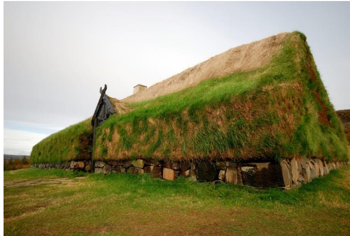
Figure 3.16. Use of green roof in Iceland [URL22]
