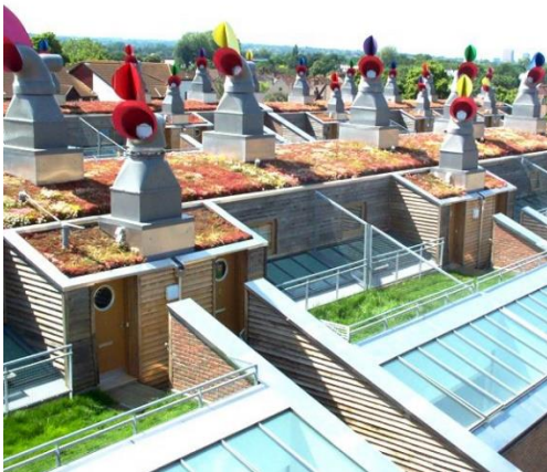
Figure 4.5. Bedzed, extensive green roof [URL75] Figure 4.6. Bedzed, windcatchers [URL76]
