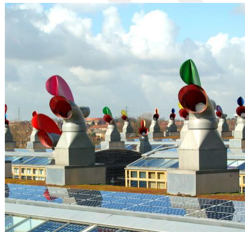
Figure 4.5. Bedzed, extensive green roof [URL75] Figure 4.6. Bedzed, windcatchers [URL76]
