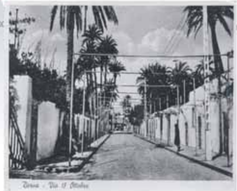
(Figure 3.49) View of street,Derna (Www.trables.com)
