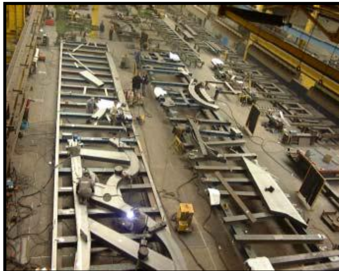
Figure 234: The sectional frames “structure” pieces welding together.
