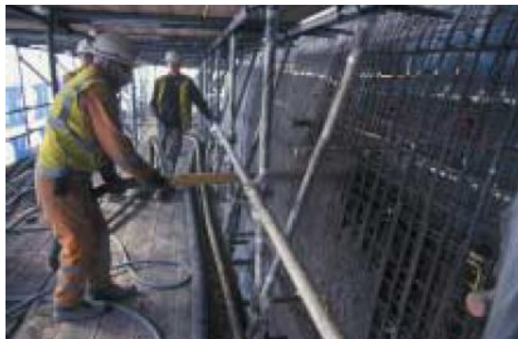
Figure 285: Spraying the substrate on site, (The Arup Journal 2005).
