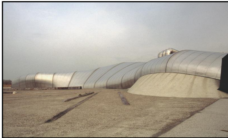
Figure 32: The exterior surfaces of the main form.
