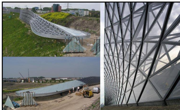
Figure 271: Real view during the construction process.
