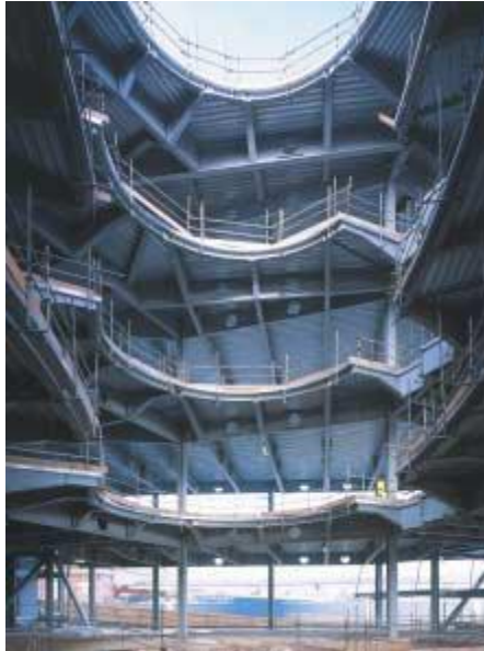
Figure 281: Atrium steelwork, (The Arup Journal 2005).
