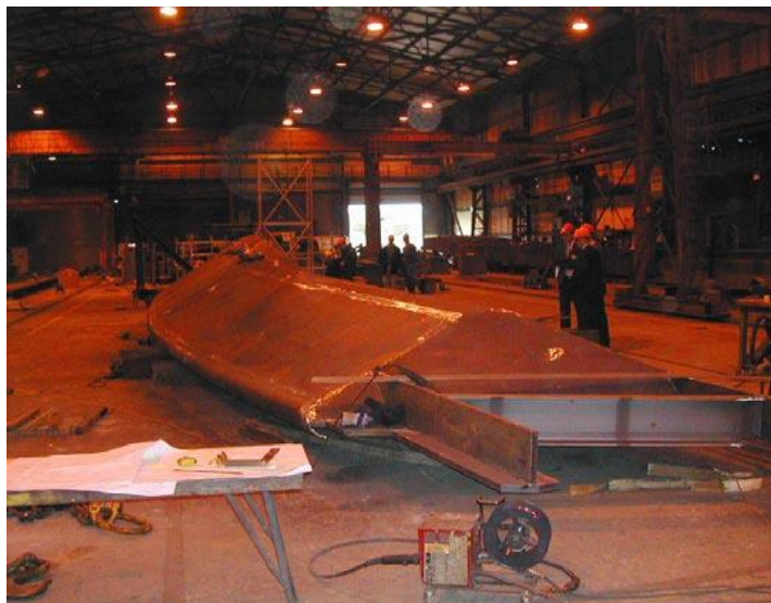
Figure 289: Pre-fabricating the bridge elements, (Michael Stacey, Philip .B and Vincent .H, 2004)
