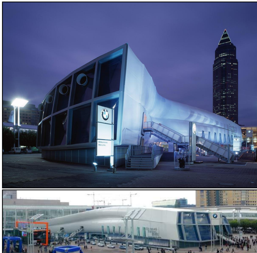
Figure 238: The completed form.
