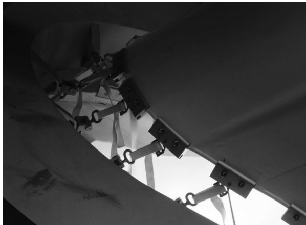
Figure 231: The outer skin of the structure.
