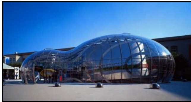
Figure 208: The BMW pavilion in Munich, Bernard Franken.
