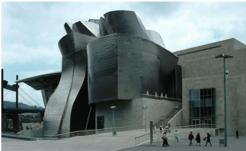
Figure 201: The types of used materials (titanium / limestone / and glass), Frank O. Gehry, 1997, (MANDOUR .A. MOHAMED, 2004).
