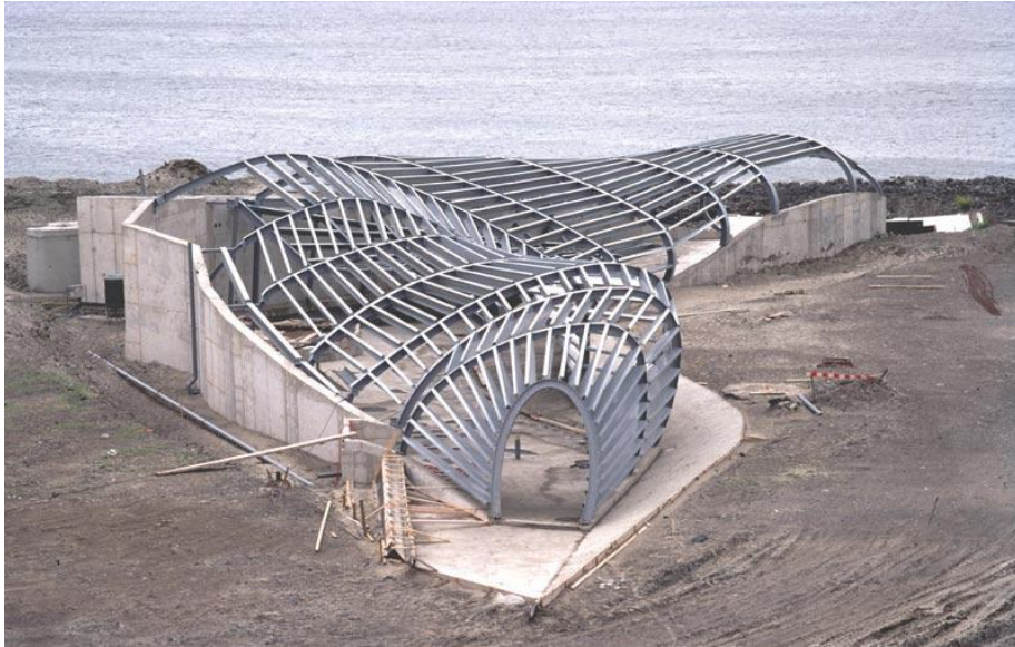
Figure 248: Wireframe steel structure of Water pavilion.
