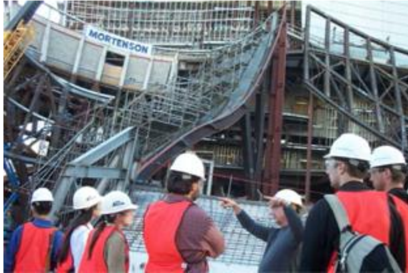
Figure 206: The building during the construction stage.
