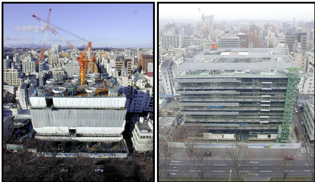
Figure 259: Constructing the façades of Sendai Mediatheque
