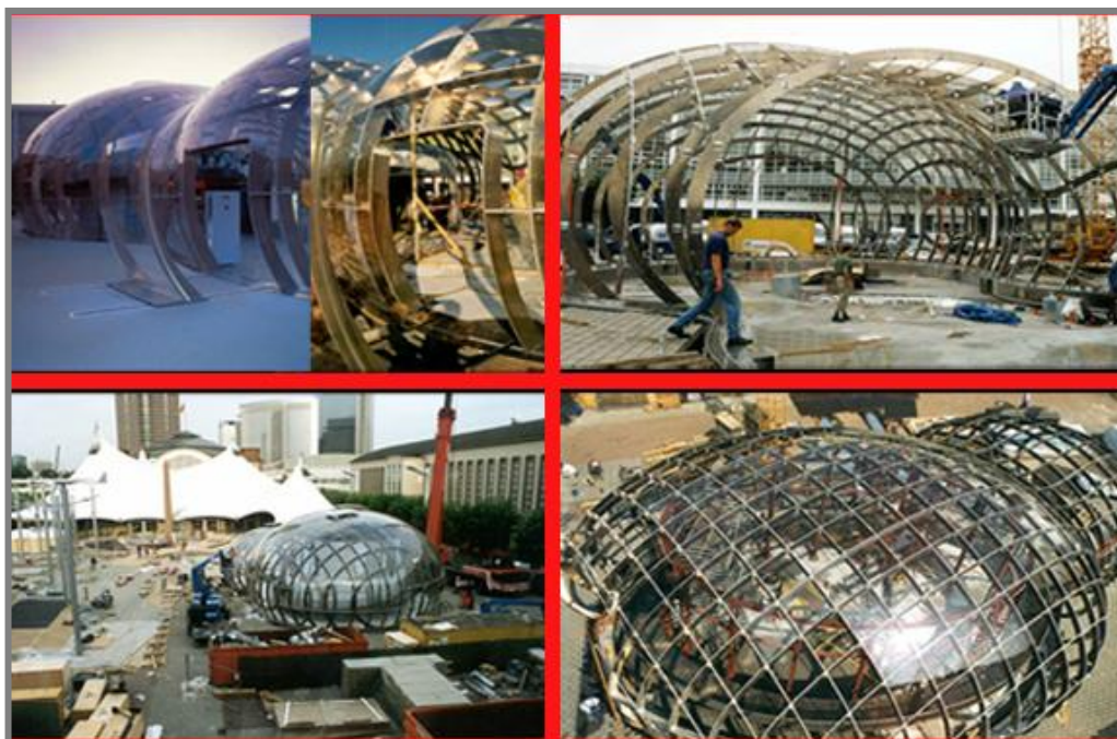
Figure 223: Finishing the final details.
