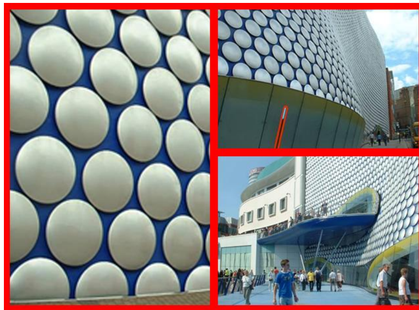
Figure 287: façade details and the Glazing at terrace-level entrance, (The Arup Journal 2005).
