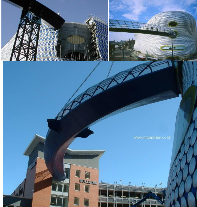
Figure 290: Completed bridge of SELFRIDGES BIRMINGHAM, (The Arup Journal 2005).
