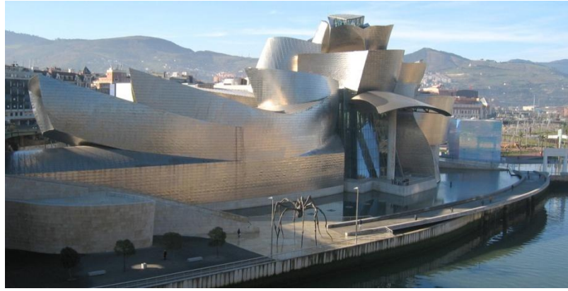
Figure 191: Frank O.Gehry, Guggenheim museum, 1997, river façade (Irene Nero, 2001).
