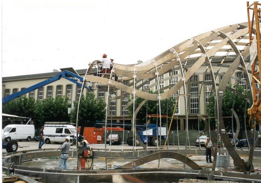
Figure 222: Collecting the structure frames.
