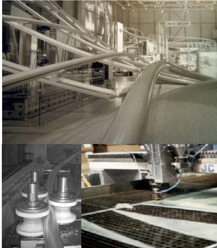
Figure 220: Cutting, twisting, and bending the structure frames. (Source: http://lapa.epfl.ch/downloads/programming_as_design_method.ppt .)
