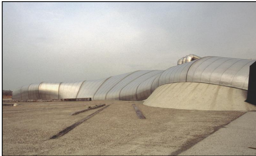
Figure 239: Water pavilion or H2O Expo exterior view.
