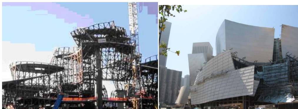
Figure 205: Collecting the pieces at the site.
