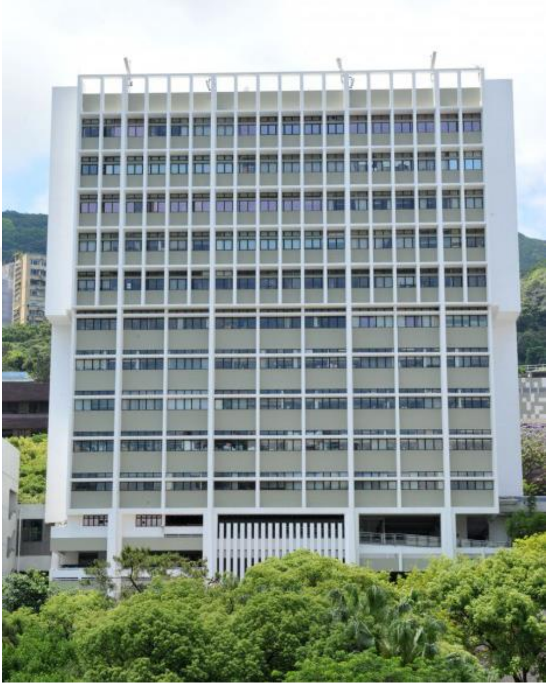
Şekil 77 Knowless Building (Estates Office, 2018)
